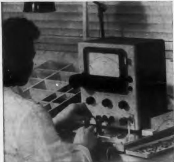
THE BRUSH Deviation Test Bridge streamlines repetitive testing of electrical products or components where resistance, inductance, or capacitance are to be measured. A large easy-to-read interchangeable scale indicates percentage deviation of impedance and phase angle deviation in radians of the test unit
