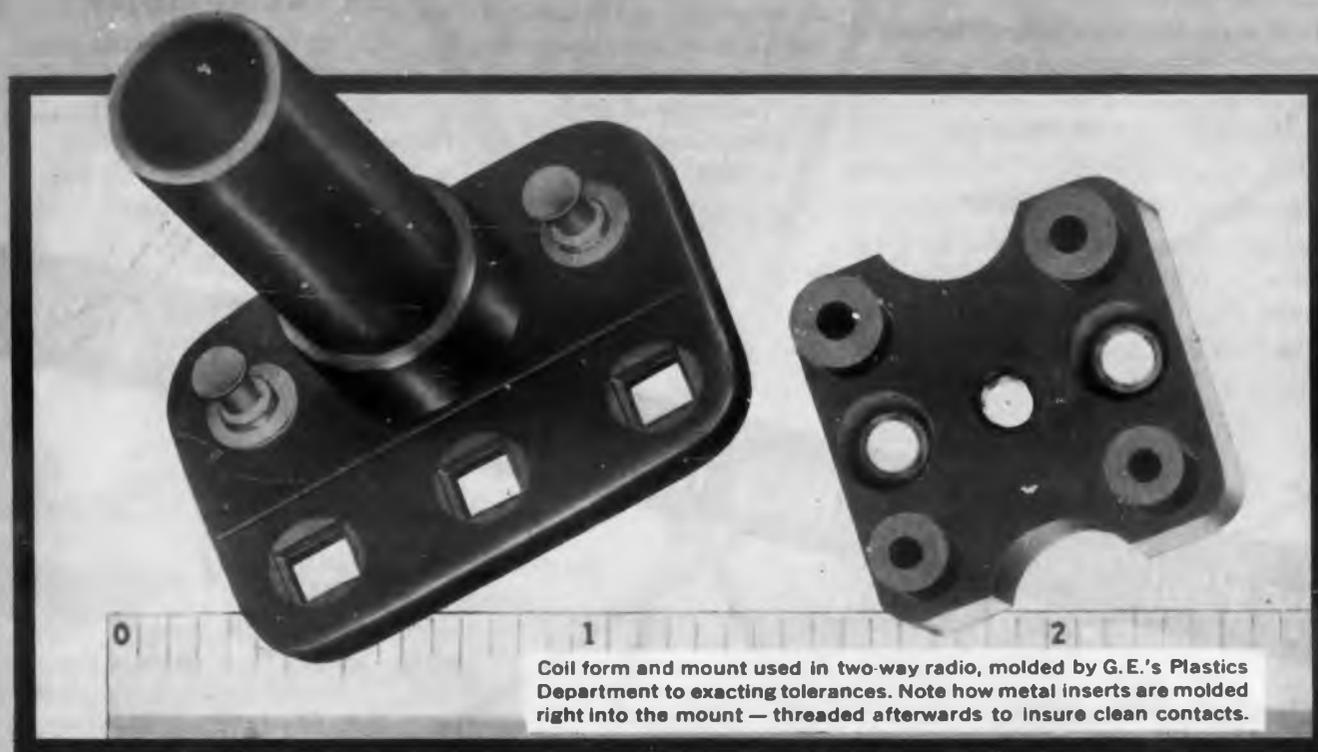
Coil form and mount used in two-way radio, molded by G.E.'s Plastics Department to exacting tolerances. Note how metal inserts are molded right into the mount — threaded afterwards to insure clean contacts.
