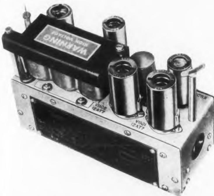
Fig. 6. Eight-watt dc input reluctance amplifier, Model 1124.
