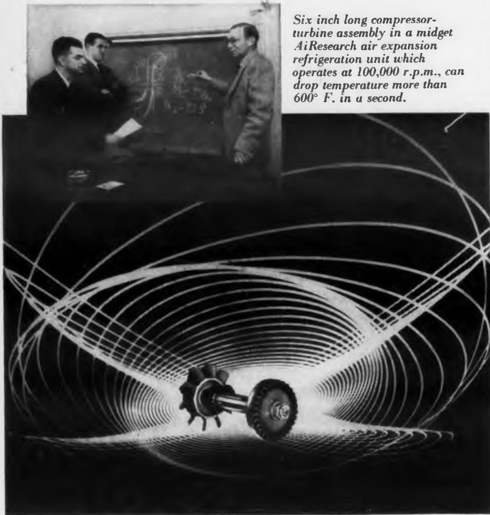
Six inch long compressor-turbine assembly in a midget AiResearch air expansion refrigeration unit which operates at 100,000 r.p.m., can drop temperature more than 600° F. in a second.
