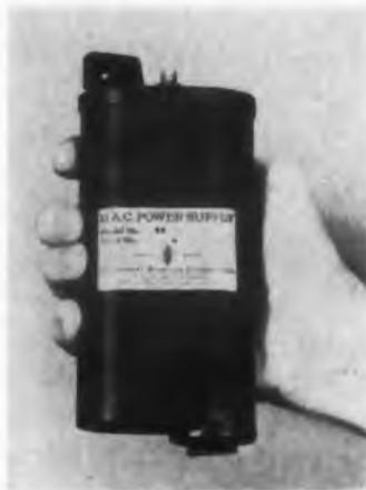
This compact, completely electronic transistorized dc to dc power supply produces 16,000 1 from as little as 3 v input. It weighs only 1-1/2 lb and is only 1-1/2" x 3" x 6". Units are also available that deliver 16 kv at as much as 200  $\mu$ a from 12 v input, where more current is desired.
