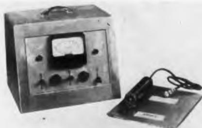
Model A-116 "Monitor" Count Rate Meter is a line-operated unit designed for quantitative radioactivity measurements. An integrating rate meter, it provides instantaneous audible and visual indications of the counting rate of radioactivity detected by the probe-type detector heads. Its stabilized high voltage supply permits use with Geiger counters, as well as with scintillation and proportional counters having built-in cathode follower or preamplifier circuits.
