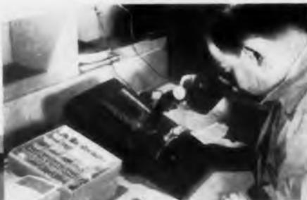
Hermetic terminals on microscope check.
