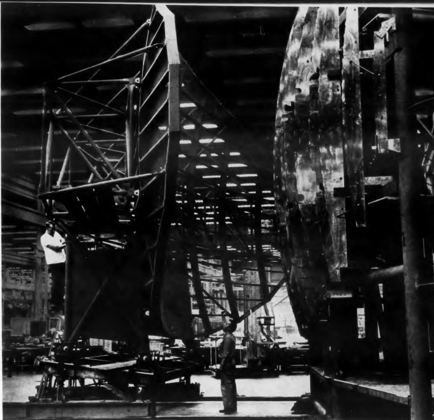
PRECISION JIG (RIGHT) GAGES ACCURACY OF HUGE ANTENNA SURFACE TO 1/100 OF AN INCH—PROOF THAT LARGE OR SMALL . . .
