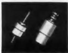
To withstand the shock, vibration and extreme temperatures involved in acceleration to 18,000 m.p.h., Chemelec (TEFLON\*) Stand-off and Feed-Through Insulators were selected for use in the 10-pounds of vital instruments nestling inside the earth satellite.
