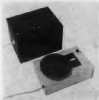
This device provides automatic positioning control for industrial applications employs an unusual application of bridge circuitry which provides positioning accuracy of 0.5 per cent and repeatability of 0.25 per cent.
