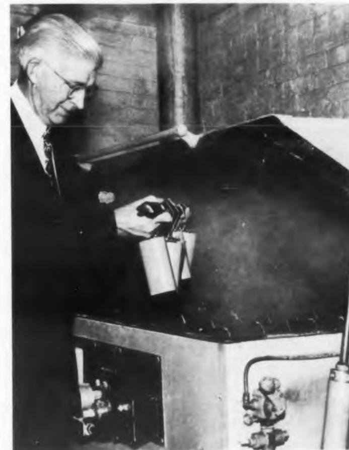
Capacitors being removed from test chambers.
