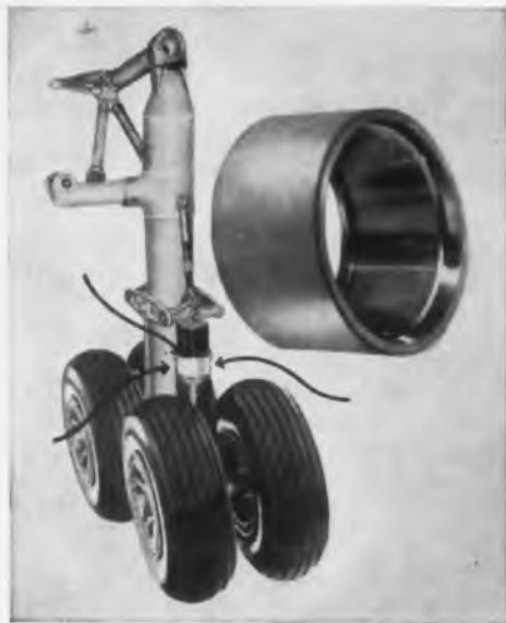
Synthane (arrow) serves as bearing in landing gear shock struts.
