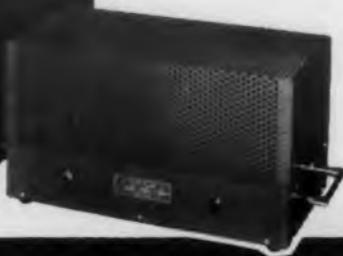
Engineering techniques heretofore used only in large expensive test equipment have been incorporated into this new Model 2400 large screen oscilloscope which displays 12 complex wave-forms simultaneously. This instrument is currently being used in the following applications: Telemetry, Stress and Strain, Vibration, Analog Computers, Medical Wave-forms and Production Testing of Multiple Circuits of Complex Studies.
