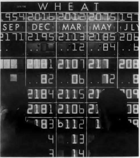
This typical application of the Hupp "Data-Tab", lighted by 2,300 G-E 2-pin lamps, posts wheat prices. It can easily be adapted to deliver practically any message—instantly.
