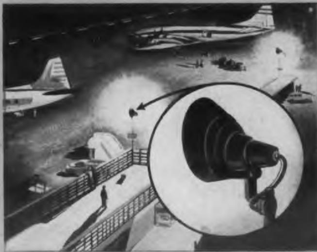
**SPECIALTY FIXTURE WIRING**—Non-flammability, resistance to heat, moisture and aging of TFE resins assure reliable performance of floodlights, heat lamps, outdoor lighting.
