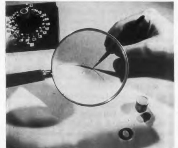
Shift register transistor is expected, with further development, to perform functions that now require a circuit arrangement of twenty transistors, forty resistors, and twenty capacitors. Object at upper left is a testing unit for the device. At lower right are elements of capsule in which an experimental unit is enclosed for testing.
