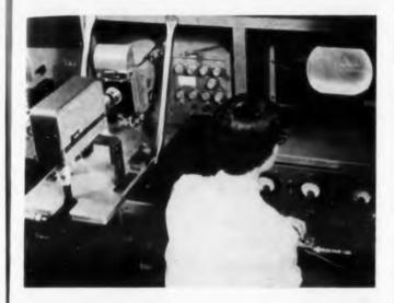
**Operator checks** transistor waveforms on television screen as part of production line inspection.
