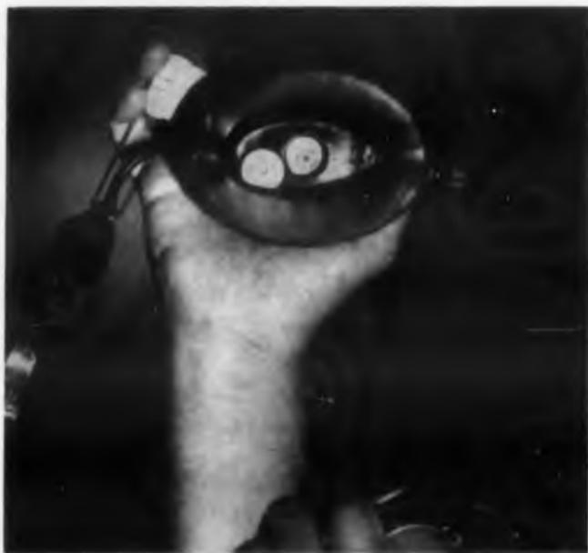
**Experimental earphones** contain a tiny circular microphone (lower disc) which picks up noise that leaks through ear cushioning. It then produces a second noise opposite in phase to first which cancels the first in large measure, and produces an artificial quiet.
