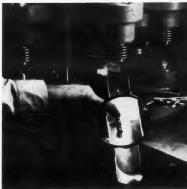
Mass production of glass inner terminal units for electron tubes is possible with the 13844 8-position, 8-head automatic sealing machine. Besides completing the glassing sequence, the machine positions a pin. Normal production is 480 units per hour, but the machine can produce 1700 units an hour if parts can be loaded that fast.
