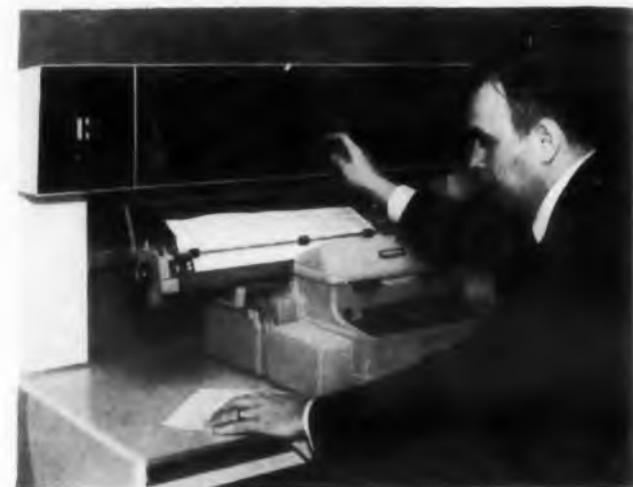
Input control console of Daystrom Systems' solid state computer, controlling 350 point alarm-scanning system at the new steam electric station of the Louisiana Power and Light Co., Monroe, La.
