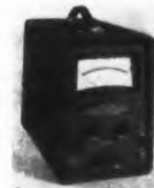
Model 5900 constant current source can be used to test semi-conductors, thermistors, clutches, magnetic cores, and other current sensitive devices. Output is 0 to 100 v, 1 to 100 ma. Line regulation is 0.5 per cent and load regulation is 0.25 per cent.
