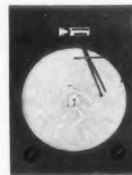
These temperature recorder-controllers cover the full range of filled systems. Model 7815 is a single pen recorder; models 7816 and 7817 are two pen, two control and one control units. Charts are 12 in., and ranges are between -100 and +100 F. A universal controller can be used for proportional, on-off, or differential gap control.
