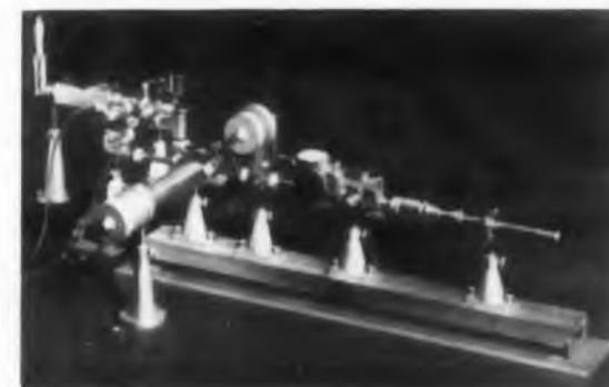
These Hilger & Watts waveguide components are for use in Q and Ka bands. The Q band equipment includes mechanically tuned reflex klystrons, swr indicators, wavemeters, thermistors with mounts, and precision attenuators.
