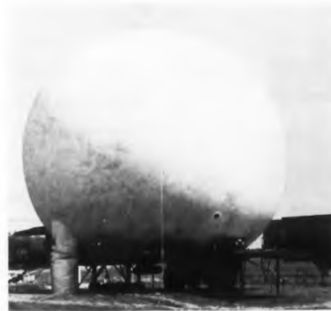
Plastic balloon , resting on mobile trailer bed like a golf ball on a tee, forms housing for antenna of Frescanar.
