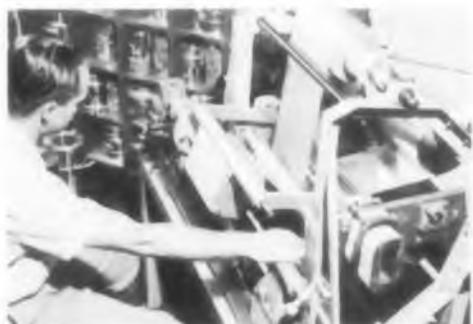
Interleaving sheet-type insulation with aluminum strip.
