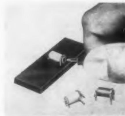
The Press-Fit SKT-103 PC miniature jack mounts flat against a printed wiring board. It has a double-prong steep strap in front, and a connection lug in back which fit in three small holes forming a triangle in a grid coordinate layout. It is dip soldered from the underside of the board for mechanical and electrical requirements. Made with a self-aligning Teflon hole, the unit takes a 0.08 in. probe with no strain on the contacts.
