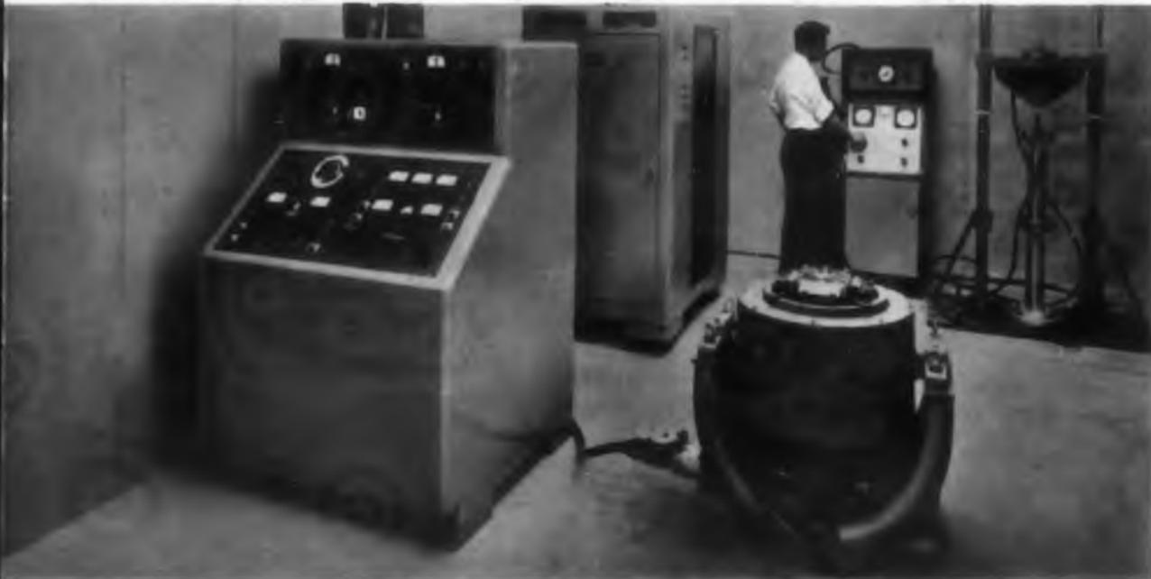
High power vibrator and "high shock" test equipment enable Ohmite to develop components for the most severe military applications.
