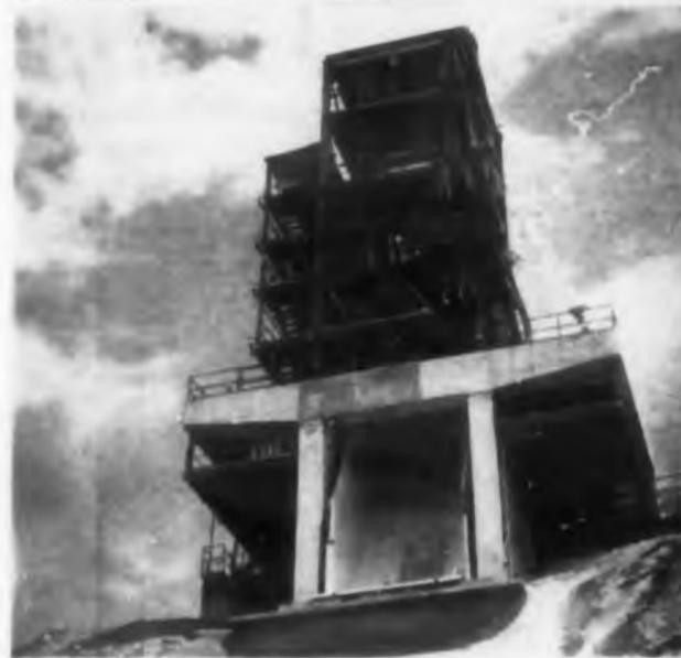
One of Lockheed's test stands with dynamic thrust mount to simulate flight environment.
