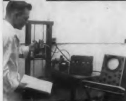
**LEAK DETECTION TEST** subjects components to minute inspection of hermetic sealing with a mass spectrometer type leak detector.
