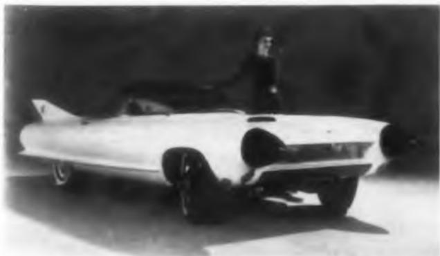
Note nose cones which house part of the experimental proximity warning device.
