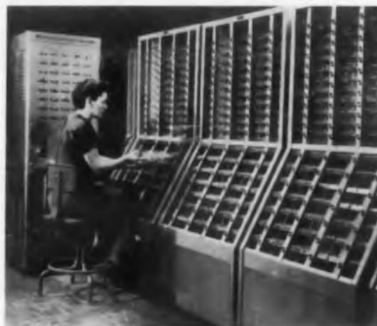
An operator removes a tray of transistors from the "honeycomb" bins of an automatic tester-sorter.
