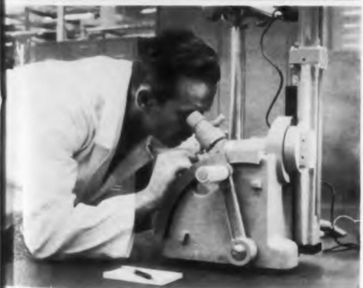
Optical gauge determines measurements within 5 millionths of an inch.
