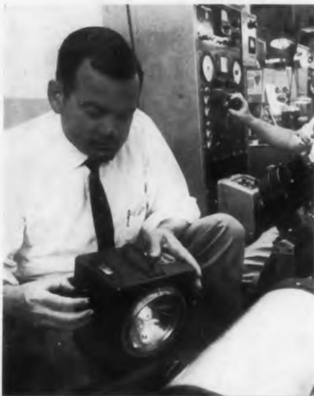
Temperature problems are part of the packaging problems Bill Rands has been solving for the past 3 years. In his work with Minneapolis-Honeywell's Aero Div., he worked out a rather simple, direct method of determining what happens thermally inside a piece of equipment. With the advent of mach 3 flight and reentry temperatures, his mockup method may well become a common procedure in designing cooling systems.
