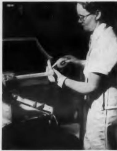
**TEFLON** Coated Glass. Coated on one or both sides. Exceptionally tough, resilient and abrasion resistant. Good electricals, chemical resistant. Very low power factor. Heat resistance up to 250 C. For coil wrappings, cable wrapping, high temperature lead wrapping on electronic gear, motors, transformers, generators.
