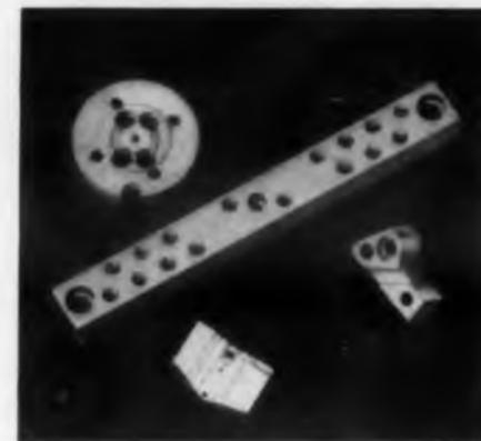
A machinable ceramoplastic insulation material Supramica 620 will operate at temperatures up to 1550 F with complete dimensional stability. It has a dielectric strength of 250 v per mil and an arc resistance of 300 sec. Loss factor is negligible. The material is resistant to nuclear radiation, will not carbonize, and can be machined to tolerances of 0.0001 in.
