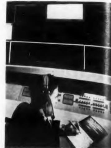
Console houses five vhf radio telephone circuits for broadcasting tide and weather data.
