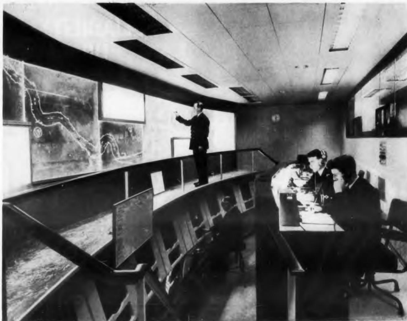
Operations room of the new Thames Navigation System at Gravesend, England, houses radar display of ship traffic, (only one of seven screens is now installed) vhf radio-telephony links with traffic, and readout of tide and visibility recorders.
