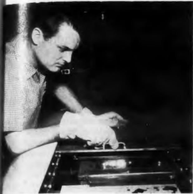
**Manufacturing engineer** checks flow solder device used in manufacture of computers in Phoenix, Ariz. A flowing river of molten solder gives a uniform, dross-free, quality connection. An advance beyond hand or dip soldering, this process eliminates touch-up and improves both productivity and quality.
