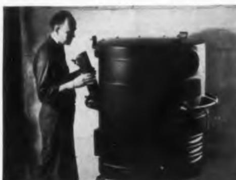
ASSEMBLY involves attachment of doors, hardware, other components using riveting, bolting, welding.
