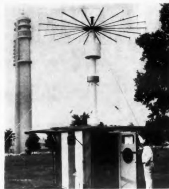
Portable version of CADF direction-finding system functions in both vhf and uhf. Roof of shelter is part of uhf counterpoise.
