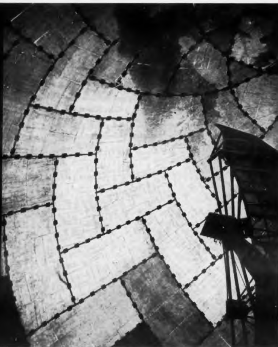
Looking upward from the inside of the world's largest stressed skin sandwich radome built of translucent fiberglass panels, securely joined by hundreds of DUAL-LOCK fasteners.
