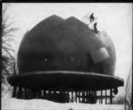
Radome designed and built by Long Sault Woodcraft Limited, St. Andrews East, Quebec, for the United States Air Force RADC.
