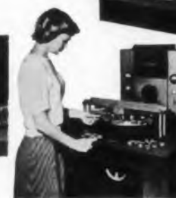
Automatic Production Unit
