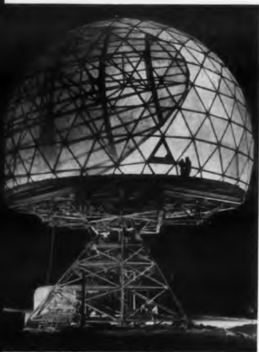
Geodesic radome is under test at General Electric's HMED facility. Bliss-designed dome silhouettes multi-beam AN/FPS-7 antenna.
