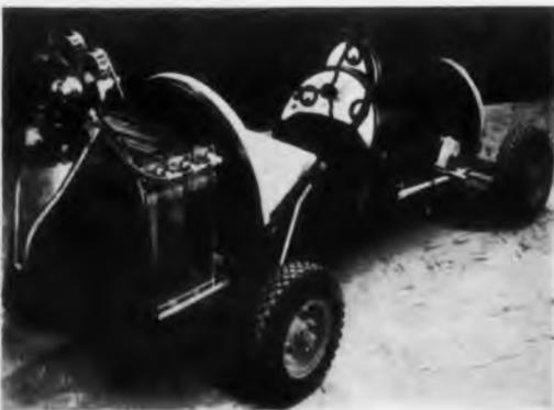
**A prototype zinc-oxygen fuel cell is the power source for this racer. Tank in rear contains oxygen which is admitted under low pressure into the cell where power is produced by oxidizing zinc fuel in potassium hydroxide electrolyte. The cell will be developed first for electric industrial trucks. After testing, it might be adaptable to automobiles and trucks.**
