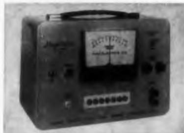
For use with rf signal generators and vacuum tube voltmeters, the Megavolter rf voltage calibrator obtains readings of 1% accuracy to 10 mc, 2% to 50 mc, and 3% to 200 mc. It measures from 1 mv to 1 v rms over the frequency range of 1 kc to 200 mc. The input impedance is 50 ohms, constant.
