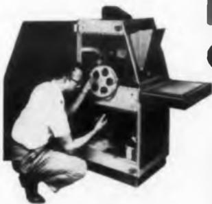
Design characteristics of EMCOR standard cabinets allow for easy accessibility to all electronic equipment and instruments.
