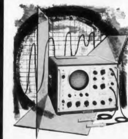
The Hewlett-Packard Company has developed a sampling oscilloscope that has a rise time of less than 0.7 millimicroseconds. Known as Model 185A, it is highly useful wherever pulse analysis of fast circuits can speed engineering, research, design, or performance testing.
