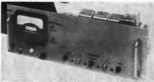
The Regohm meter relay can be activated by signals as low as  $2 \mu\text{w}$  and can control up to 600 w of output power. For use in process control, the unit can be driven from low-level electrical signals, or the output of differential transformers, strain gages, gas analyzers, bridges, temperature-sensitive elements, or photocells. The output of the relay is available for sequential operation of up to nine power relays and for stepless control of wattage.
