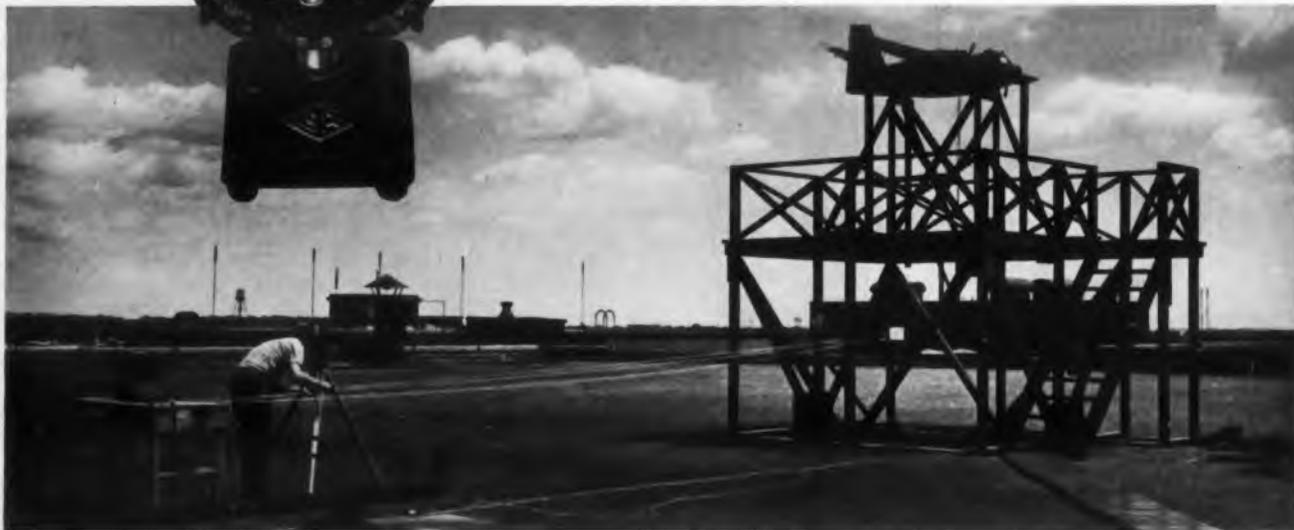
A tribute to the Admittance Meter's versatility is its use at Grumman Aircraft, Bethpage, Long Island. Grumman engineers were faced with the problem of making accurate measurements on developmental aircraft antennas without influencing, by their physical presence, the antenna's radiation pattern or impedance characteristics. As a solution, they mounted an Admittance Meter, a
