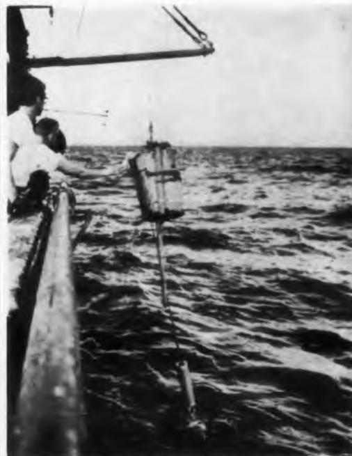
**Ocean-bottom seismograph**, developed by Lamont Geological Observatory, gets its first test (above). Acoustic telemetry package is strapped to trash barrel containing batteries. Seismograph itself is suspended from the can. At right, Chuck Hubbard, Lamont engineer, tests improved version to be used this summer. Metal cylinder on lab bench is moving coil geophone. Magnetostrictive pinger sings away merrily in oil drum behind Hubbard. Operating scheme is shown in block diagram.
