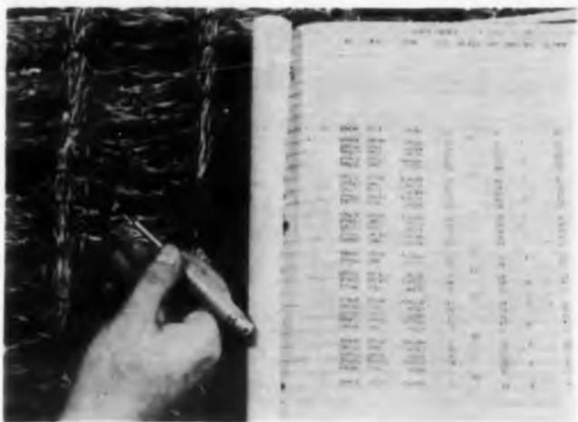
**Wiring list** at Litton's Electronic Equipments Div. makes it easy to wire new computers, obviates wiring diagrams.
