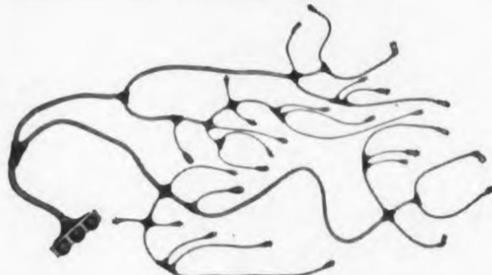
General Electric silicone rubber used extensively by Aerojet-General Corp. for the Titan ICBM's propulsion-system wiring harness. Break-outs and junctions molded from G-E RTV, wiring is silicone insulated, jacketing is high-strength G-E silicone rubber — all chosen for their stable insulating properties, resistance to temperature extremes and weathering, and stability in storage for many years.
