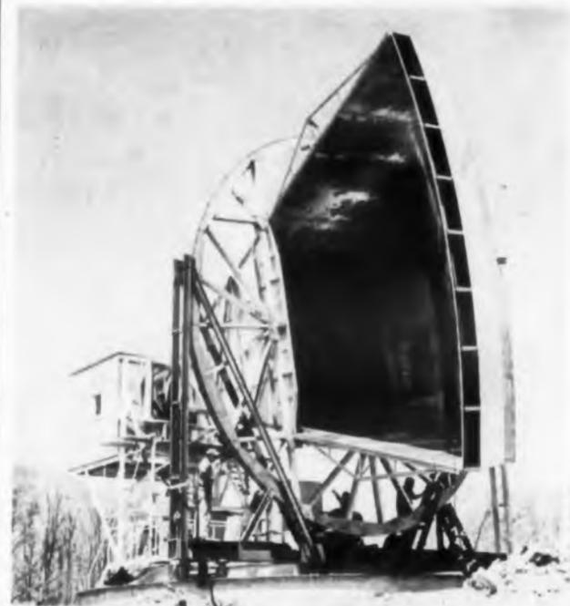
**Parabolic horn antenna** at Holmdel tracks Echo with minimum thermal noise. "There seems to be little room for improvement insofar as noise is concerned," said one Bell Labs engineer of the big horn. Maser amplifier and other receiving gear are housed in cab at the small end of the horn.
