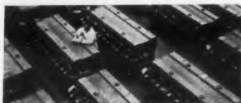
Inspecting one of Synchrotron's 240 magnets. This one weighs about 17 tons. Inconel "X" tube fits into narrowest gap between jaws.
