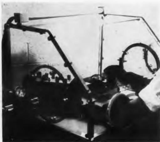
Fig. 2. Dry box provides a dehumidified atmosphere for components which are moisture sensitive.
