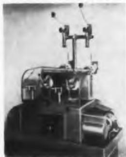
TV vertical deflection coils may be toroidally wound on the TVL 59 winding machine. Both halves of a split ferrite coil are wound simultaneously, ensuring positive symmetry of cosine winding. Resultant shorter wire lengths reduce resistance and dissipate less power. The width of each layer, and the number of layers, can be automatically adjusted. Wire diameter may be from 0.008 to 0.020 in. for winding at the rate of 400 rpm. Winding angle is 120 deg max, 15 deg min.
