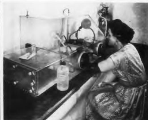
**Fig. 4.** Vacuum oven inside the air lock contains components which have been baked dry. The components are taken from the air lock into the dry box where they are hermetically sealed. Bubbles in the glass bottle indicate the air lock is being constantly purged with clean dry air.
