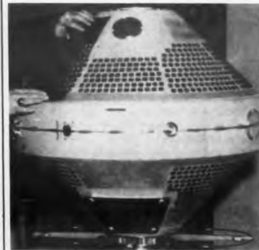
Squares of red and stripes and patches of silver paint help keep instruments in Explorer VIII comfortably cool.
