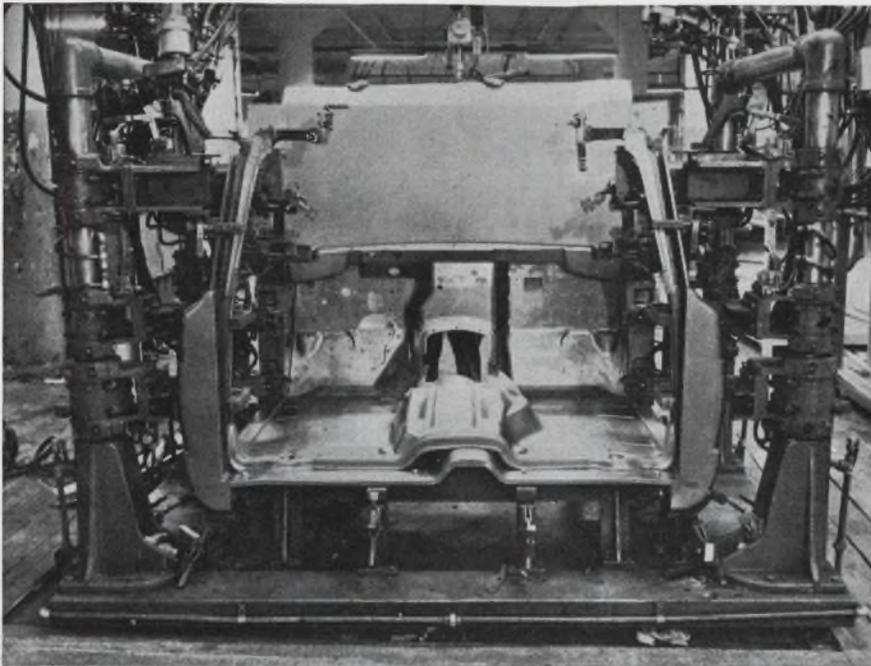
**Resistance-welding fixture** at Kaiser Jeep Corp. incorporates simplified tooling plus standardized welding equipment (paper 29.1)
