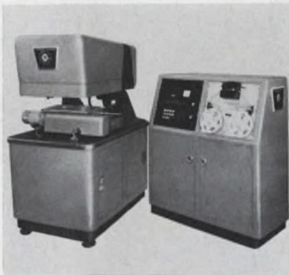
Series 15J tape controlled grid drills operate with infinitely variable spindle speeds of 10,000-50,000 rpm. The positioning table may be moved a maximum of 24-in. in both the X and Y directions. Each individual spindle is programmed to "use" or "not use" for each machine cycle. Control input is through 8-channel 1-in paper tape which can be prepared by flexowriter or equivalent means. Gardner-Denver Co., Grand Haven, Mich. Phone: (217) 222-5400.
