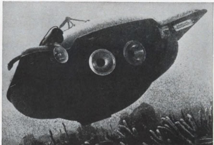
Deepstar three-man vehicle is designed to dive to a depth of 4000 feet. Developed at the Westinghouse Defense and Space Center, it will be leased for scientific dives.
