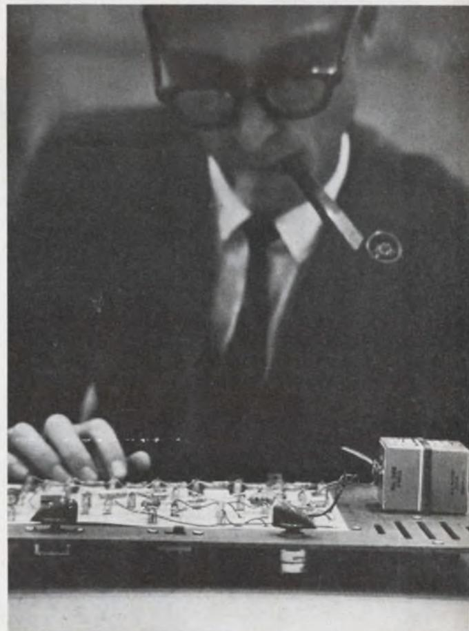
Coauthor Casazza fingers a tune on this organ, built from a Norelco electronic projects kit. Armed with transistors and diodes, the experimenter can build a number of different gadgets by plopping a wiring diagram over the spring clips and hooking away.
