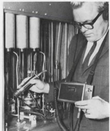
As the microphone nears a leak, an audible hiss gets louder. The leak detector also has a meter and volume control.
