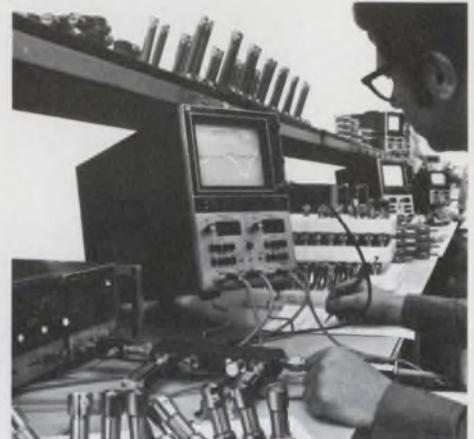
In a typical production test application, the 8755L large screen display shows forward- and return-loss response of components.
