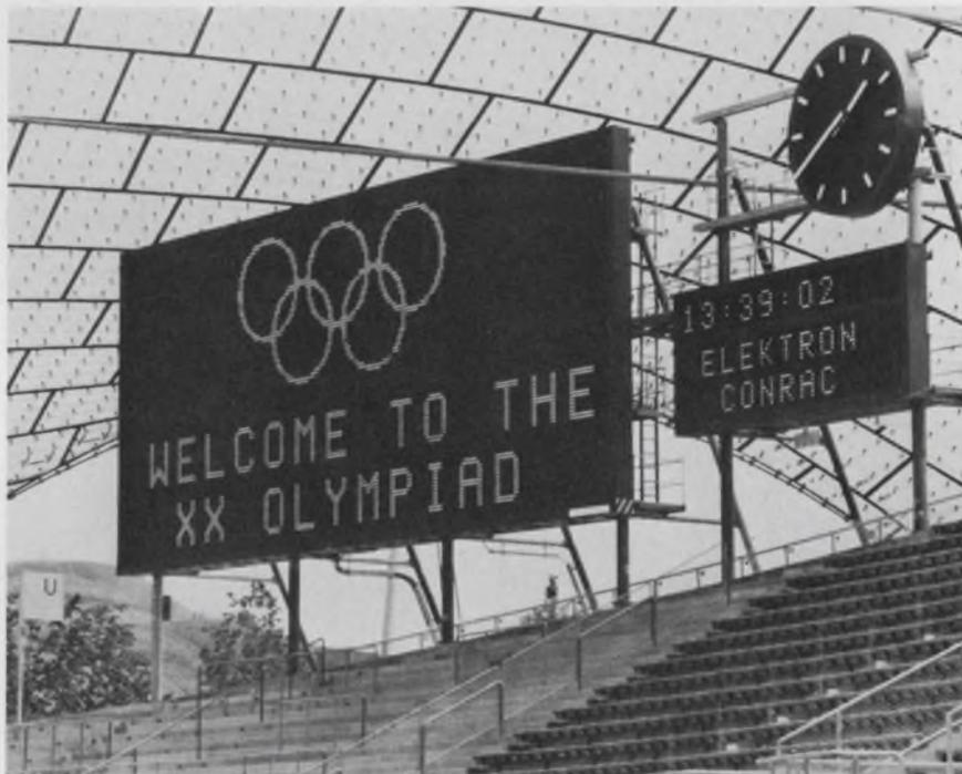
Two giant, computer-controlled displays, designed by Conrac Corp., have been installed in the Olympic Stadium in Munich, the principal site of the Summer Olympic Games. These boards use up to 1.26 MW for operation.
