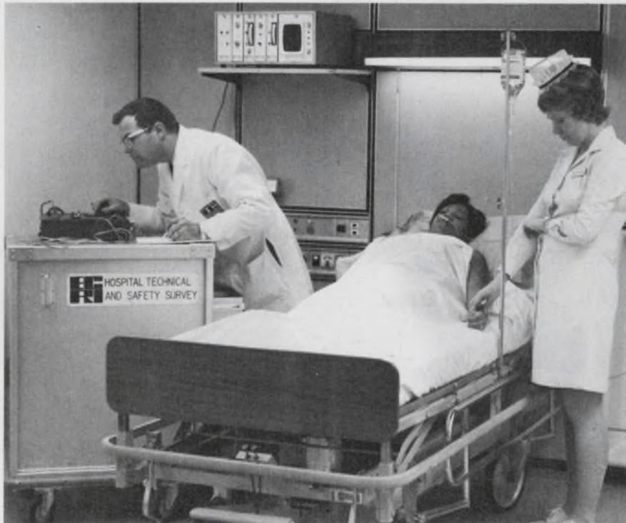
**Hospital surveys** are performed by the Emergency Care Research Institute to evaluate the efficiency of equipment. A nurse watches over the patient while equipment is disconnected for testing.
