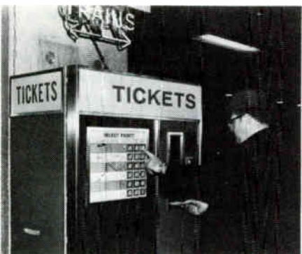
Photos Courtesy Cubic Corporation
