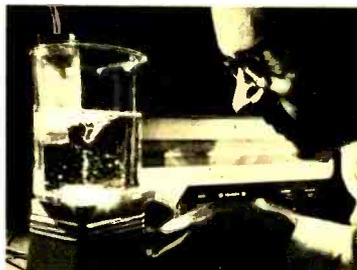
turned by a second, motor-driven magnet in the beaker stand. And the device mounted atop the modern-day caldron is a plastic-covered electronic sensor designed to measure the strength of the chlorine solution inside. Though our photo shows a prototype version, the people at Honeywell hope eventually to market their super sniffer to owners of swimming pools, water-treatment plants and other interested in getting an electronic low-down on what's what in their H<sub>2</sub>O.
