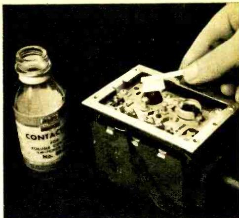
Toothbrush dipped in or sprayed with solvent makes handy tool for cleaning leakage path between closely spaced contacts. Area surrounding tube socket of TV tuner is likely candidate.
