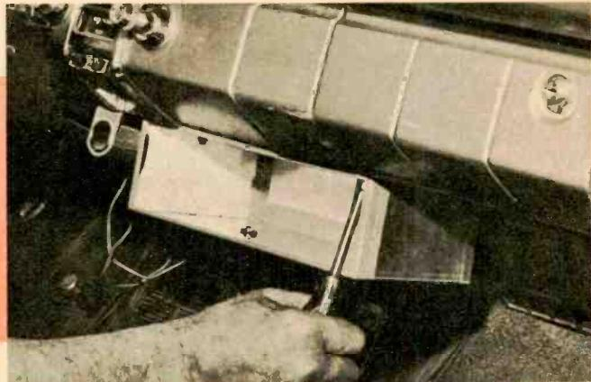
After resistor has been adjusted, install the chassis under the dash with self-tapping screws. Connect negative power lead to car chassis and positive lead to cold or accessory lug on ignition switch.
