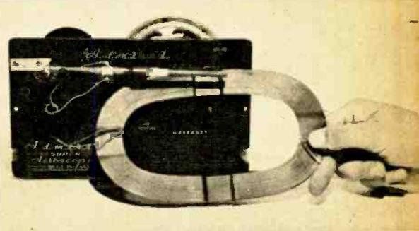
Replacing old-style loop antenna with modern ferrite rod permits addition of external long-wire.
