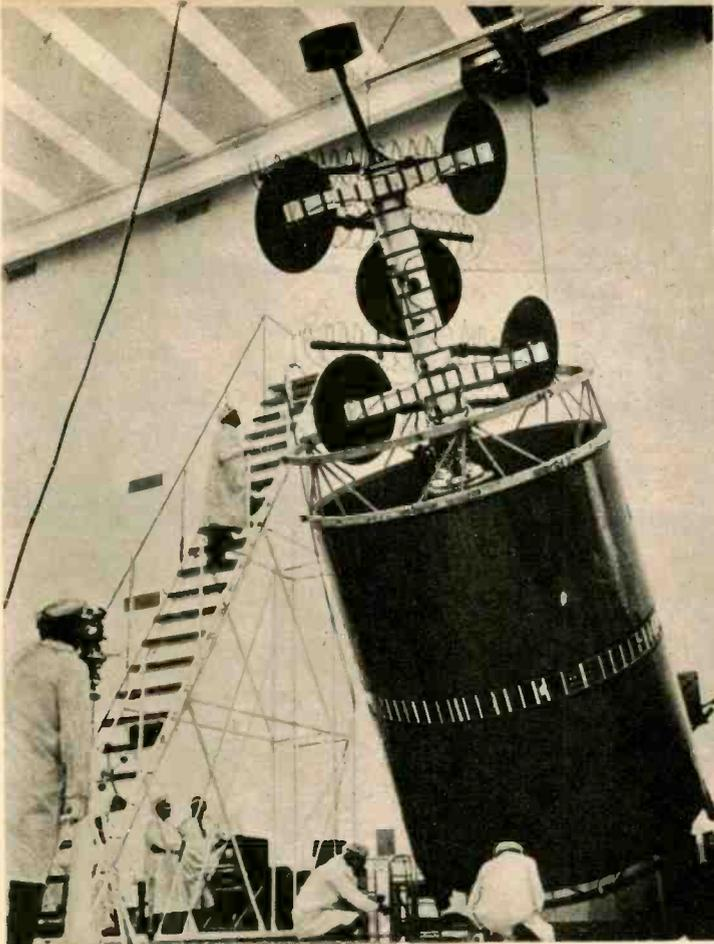
**Tactical Satellite? . . .** The Air Force Space and Missile Systems Organization now has a new baby to play with. It's an experimental communications satellite—the largest and most powerful ever—built by Hughes Aircraft. The monster is as tall as a two-story building and will be launched from Cape Kennedy into a synchronous orbit aboard a Titan-3 booster. This round fellow can handle 10,000 telephone channels and pop them into dish antennas only 1 ft. in diameter.
