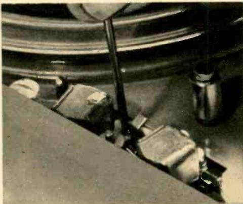
Fig. 7—On this two-head (erase and record/play) recorder, tilt-adjustment screw is on side of head. Refer to recorder's manual for location.
