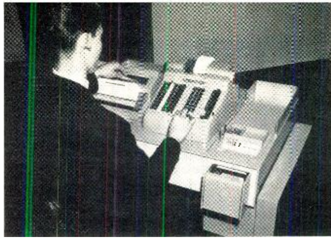
The operator is using an inscriber to imprint the dollar amount on each check in magnetic ink. Then the machines take control.
