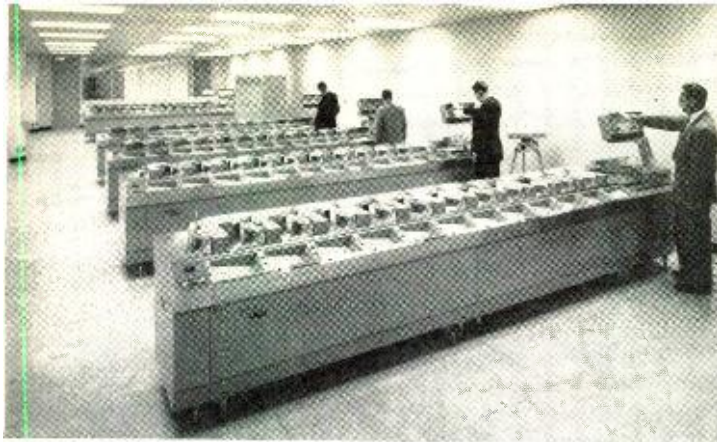
The document handling or sorter-reader section of Bank of America's Electronic Recording Method of Accounting system.
