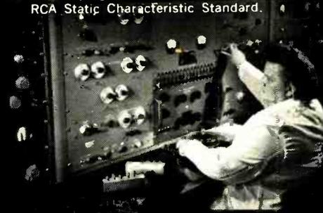
Calibrating portable Standard Cell on the RCA Primary Voltage Standard.
