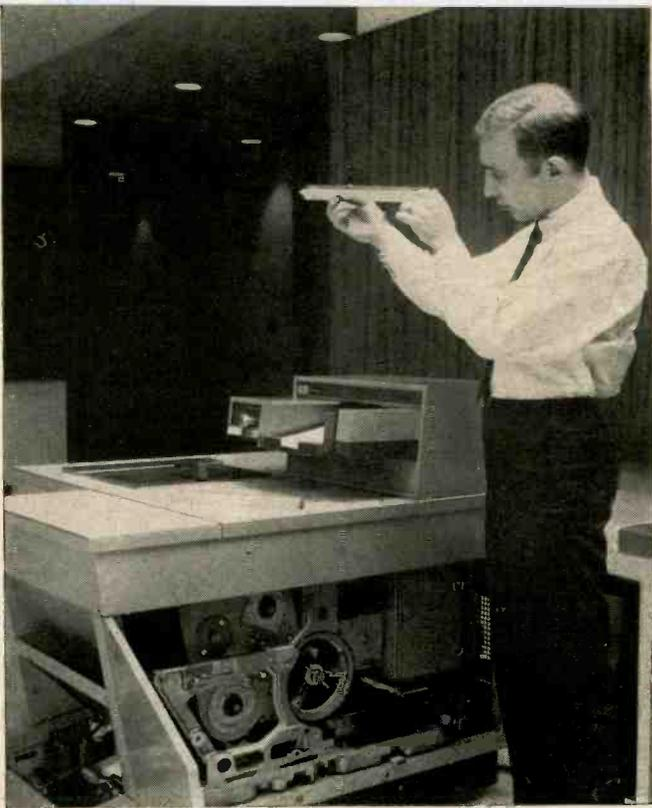
Looking for flaws in the carotron assembly used in a copier. This assembly gives the selenium drum a positive charge that prepares it to receive the electronic image.
