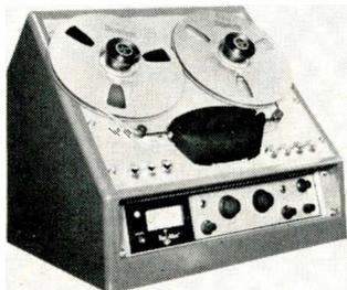
instead of the conventional single capstan, the unit has a starting time measured at less than 0.01 second and a stopping time equal to 1/2 inch of tape at 7 1/2 ips running speed. This quick reaction permits ultra-precise programming and editing, actually enabling the user to "split" a recorded eighth note.
