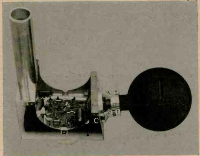
Radiation experiments carried in Mariner-IV (Mars) satellite. (Above left) Cosmic-ray telescope using solid-state detectors. (Above) Ionization chamber experiment using a five-inch stainless-steel sphere. (Bottom left) Trapped radiation experiment.
