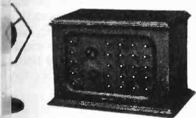
The Multi-Trol contains: Remote control for radio set; control switches for turning on or off radio, phonograph, and phone; master volume control for all speakers, etc. This unit is manufactured by the Multi-Phonograph Company, Inc., 1700 Avenue, N. W., Grand Rapids, Mich.—*Electronics, Sept., 1930.*
