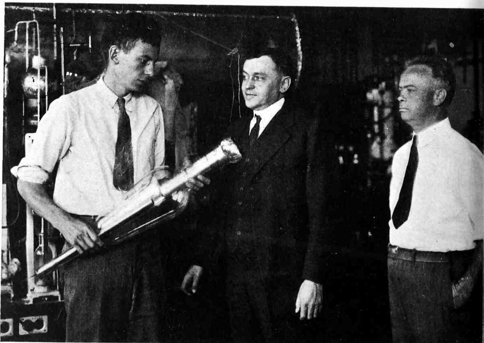
A 300,000-volt Lenard-ray tube the electrons from which are projected clear through a thin glass window and out into the open air where they may be used to bombard familiar substances, producing changes in structure and chemical combination (see pages 294 and 295). The tube is being held by Dr. Slack, inventor of its improved construction. Dr. Harvey Rentschler and Dr. Ulrey, both of Westinghouse research forces, are seen looking on
