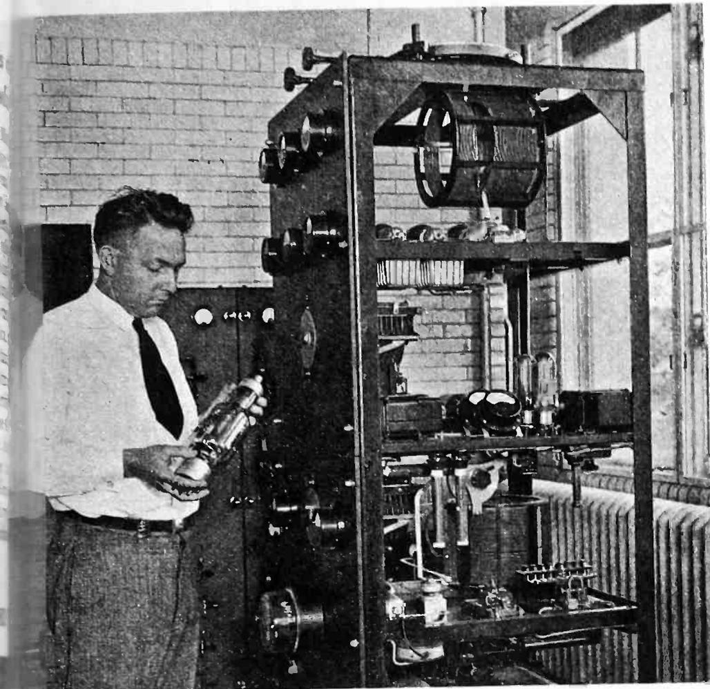
Transmitter which broadcasts half-hourly weather reports from Station WQDW, for the guidance of traffic on the airways radiating from Detroit. The operator is holding one of the ten 250-watt tubes with which the transmitter is equipped
