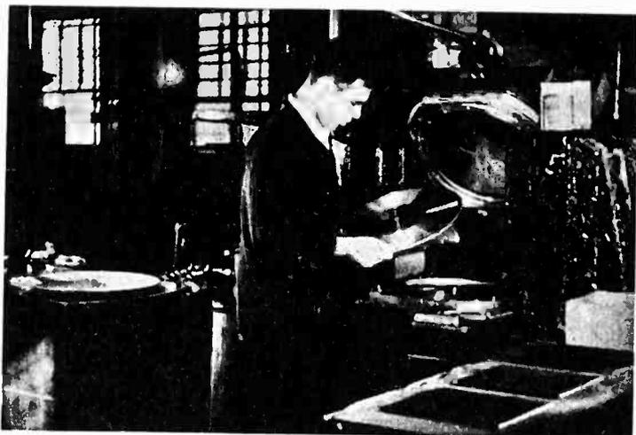
Fig. 2—Record press, showing finished record just removed from the dies, and record stock heating on the steam table
