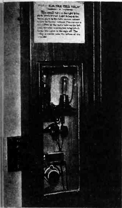
Approach of a visitor intercepts light falling on this cell, actuating sign through relay
