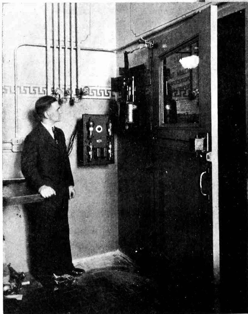
The famous "open sesame" door to the electronics research laboratories of the General Electric Company, at Schenectady, N. Y. Upon knocking the proper number of times, with intervals, a series of thyratons operate relays, and the door swings open
