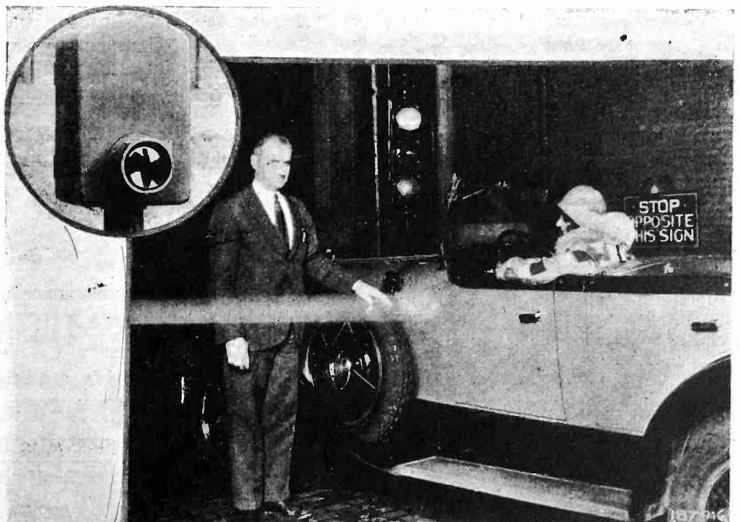
When the driver approaches a main traffic artery, the interception of the light beam shown, sets the signals to let cross-traffic go ahead
