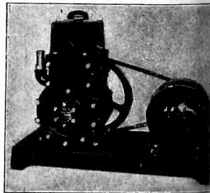
in. At a speed of 425 r.p.m. it reaches a pressure of one micron in one-fifth the time required by the Cenco Mercury Pump. The unmounted Hypervac sells at \$250, and mounted with a volt a.c., ¼ hp. motor, at \$350, f.o.b. cago.—*Electronics, October, 1930.*
