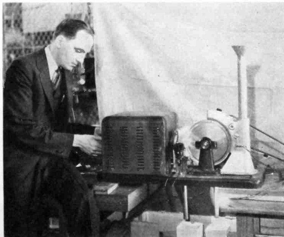
Two hundred of these photo-electric sorters are to be installed to comb over a carload of beans a day
