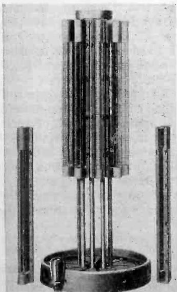
Support for the nine filament wires requiring 500 amperes of current and emitting 160 amperes
