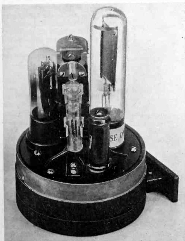
Burgess selenium bridge, triode and relay apparatus
