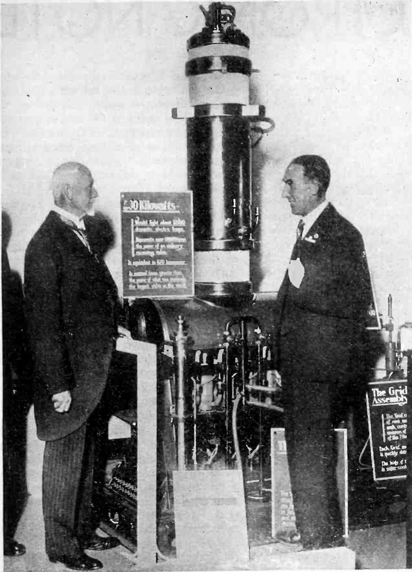
General Jan Smuts (left) and Colonel Vignoles, Electrical Association of London, inspect Metropolitan-Vickers' new continuously-pumped triode to replace a bank of tubes at the Rugby station
