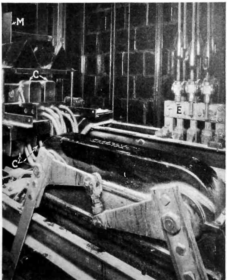
Top of one of the express cars, showing four leveling tubes at C, and one of the leveling vanes at M
