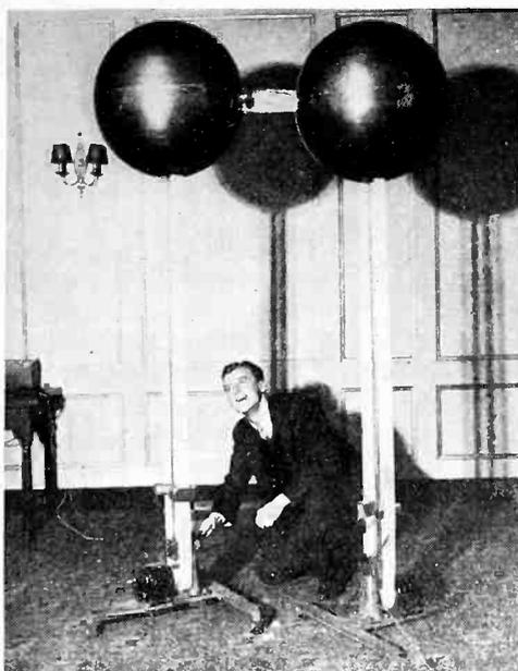
Dr. Robert J. Van Greef demonstrates his generator capable of producing 1,500,000 volts and a model of which will be used with higher voltages to disrupt atoms
