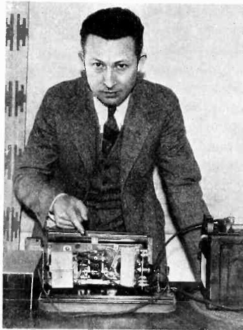
F. F. Hutchinson of San Francisco, with his power converter which steps up 6 volts d.c. to 110 volts a.c. for operation of radio sets
