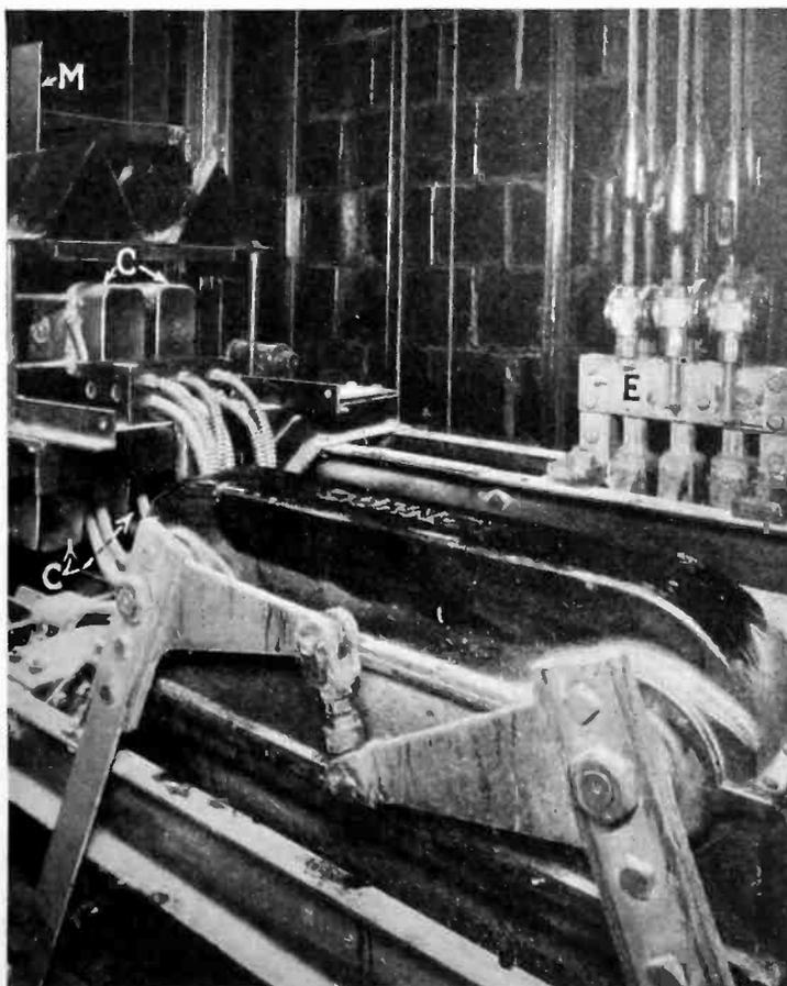
Top of one of the express cars, showing four leveling tubes at C, and one of the leveling vanes at M
