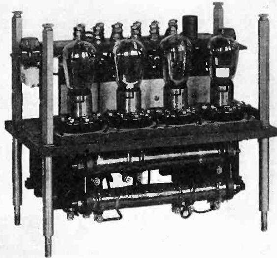
Four-tube amplifier using Pliotron tubes for cab signal equipment
