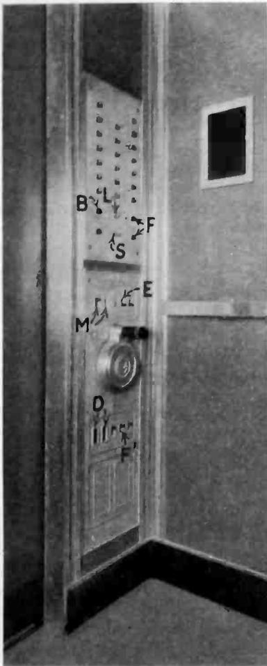
(Left)—Car-operator's lever and push-button panel
