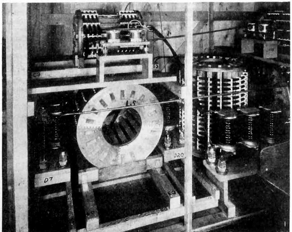
A huge completely shielded filter built at the Bell Laboratories for long-wave radio telephone research
