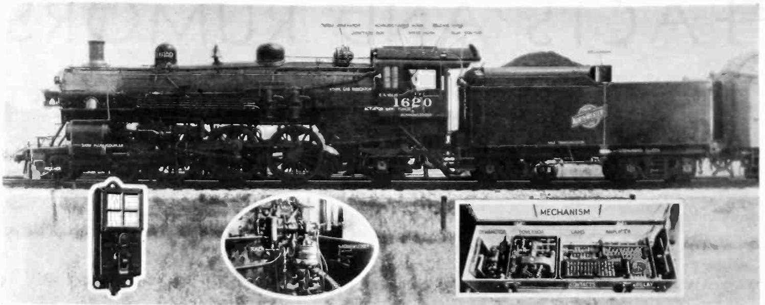
Locomotive receiving equipment designed by General Railway Signal Company showing principal component parts as installed for service use. The amplifier in this installation is mounted on the tender
