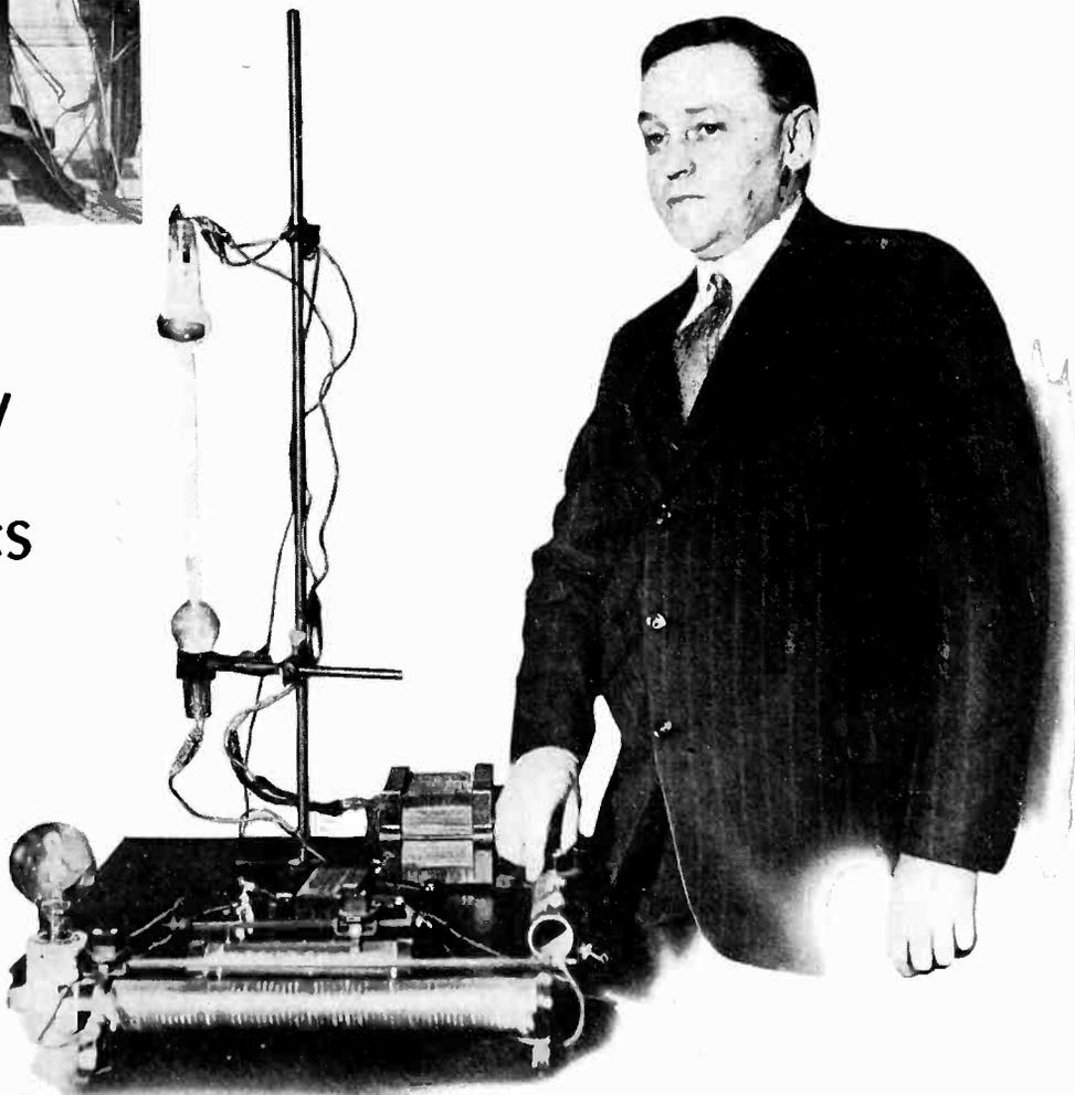
Dr. Harvey C. Rentschler, director of research, Westinghouse Lamp Co., demonstrates new sodium-vapor tube lamp which is three times as efficient as neon tube. Formerly sodium-vapor tubes quickly blackened and became useless; invention of new glass by Dr. Pirani, Berlin, avoids discoloring
