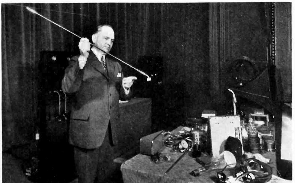
Sergius P. Grace, of the Bell Telephone Laboratories, is holding a permalloy rod in a north-south direction. In this position, due to the earth's magnetic field, the rod becomes a magnet of sufficient power to hold up a block of steel which falls when the rod is moved from its position
