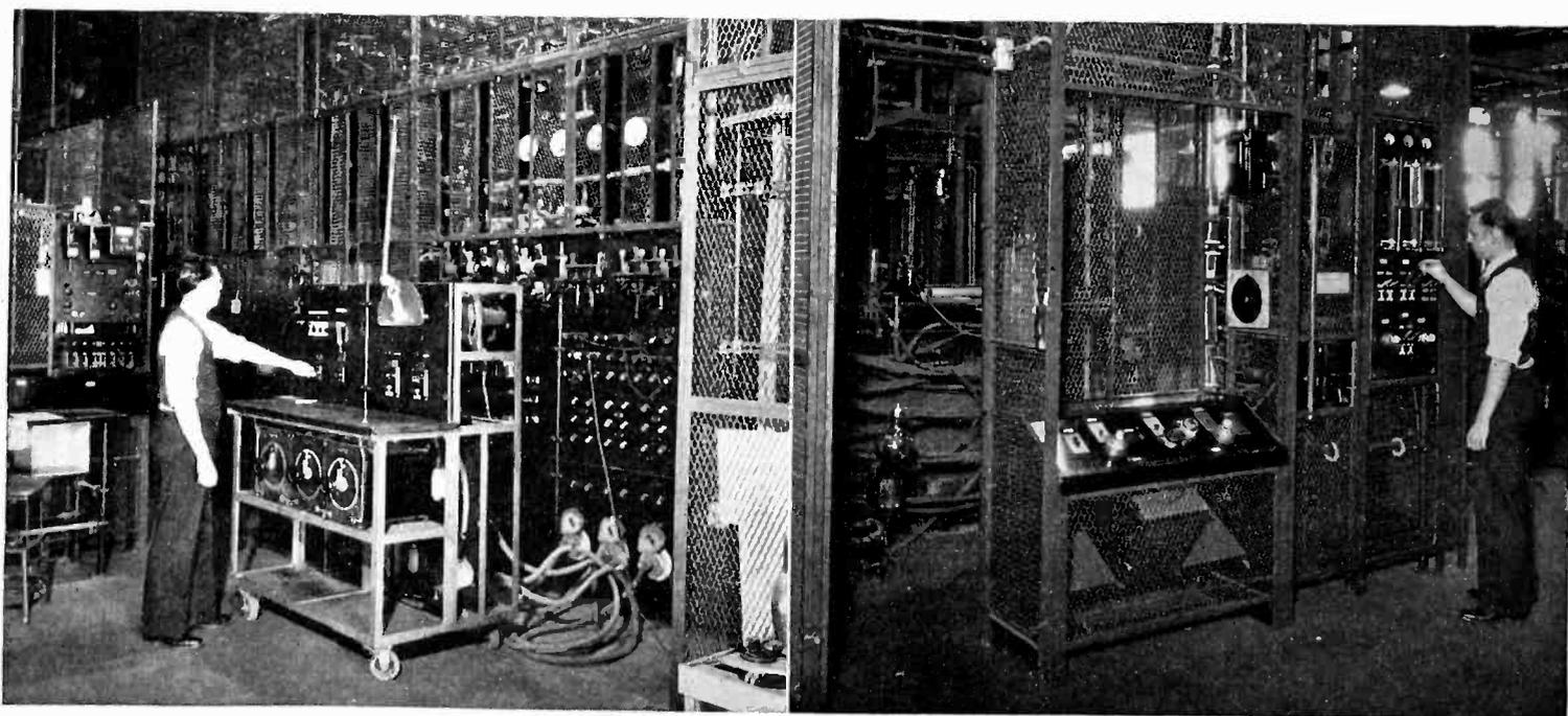
A 1,000-kva. test set. Transformers, voltage regulator and oil circuit-breakers are in other rooms
