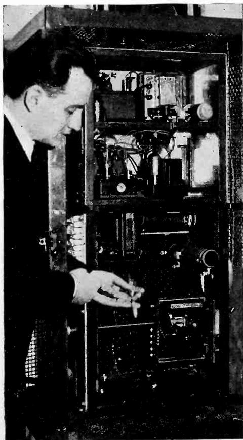
A Chicago inventor employs thermionic tubes as a fire-alarm apparatus, arranging thermo-electric couples to detect the presence of undue heat. An amplifier then sends in the alarm
