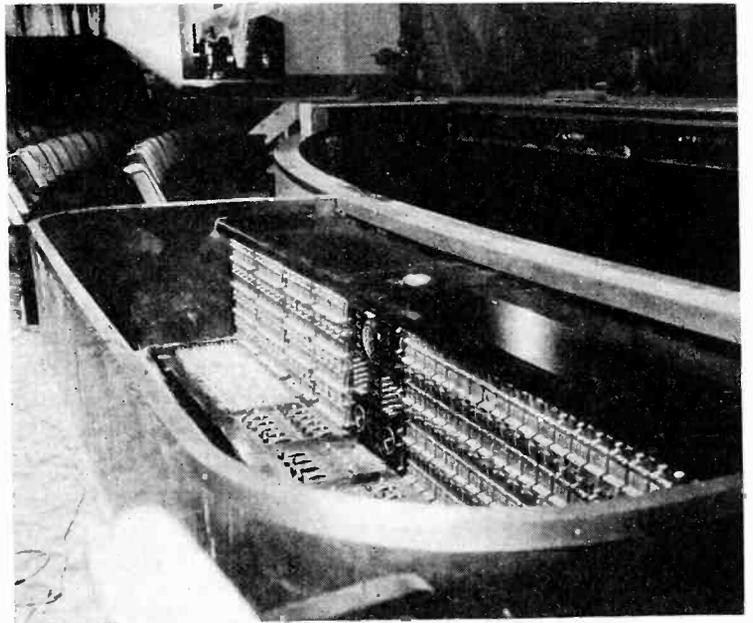
The lighting-control box in the pit of the large theater, with its 2000 control knobs
