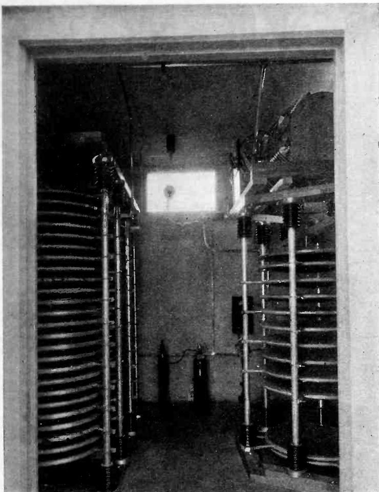
Fig. 6—Harmonic suppressing equipment in field installation of high powered broadcasting station
