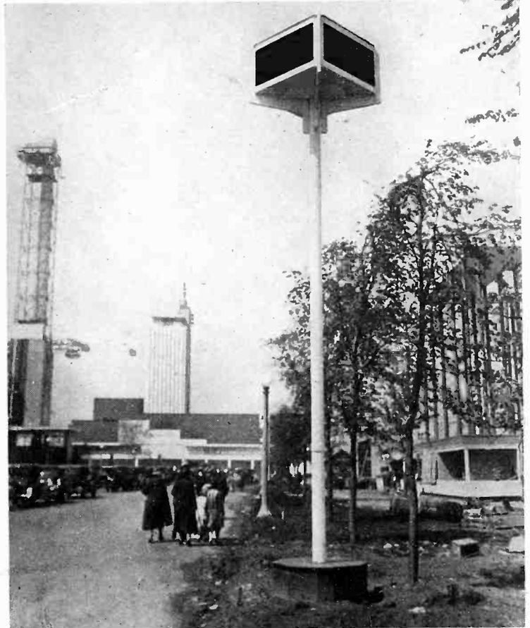
Loudspeakers throughout the grounds. Each of these 45 posts carries two speaker units, with the amplifier in the base
