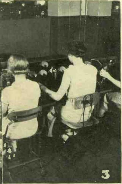
placed in bulbs. The constant concern of each operator is her "quality score". (3) A portion of the "test battery," through which every RCA Cunningham Radiotron must successfully pass before being packed for sale.
