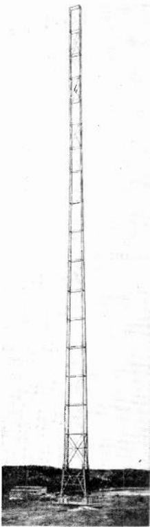
a flexible scheme of construction was developed which affords the radio engineer new tools to work with, opening up possibilities of antenna performance not hitherto possible. Self-supporting towers up to  $\frac{5}{8}$  wave for the complete range of broadcasting frequencies, are now economically feasible.
