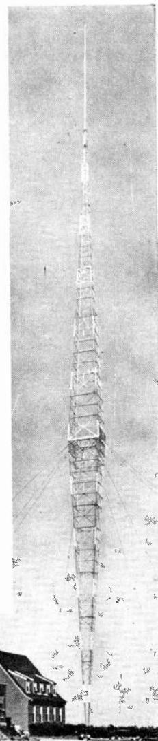
WLW's double-taper tower. Increases in signal strength up to 40% were reported when it was installed.
