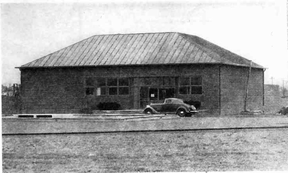
The completed station building. Note the complete absence of any overhead conductors leaving or entering the station. Buried power lines, telephone cable, and an underground r-f transmission line to the antenna make this neat-looking installation possible
