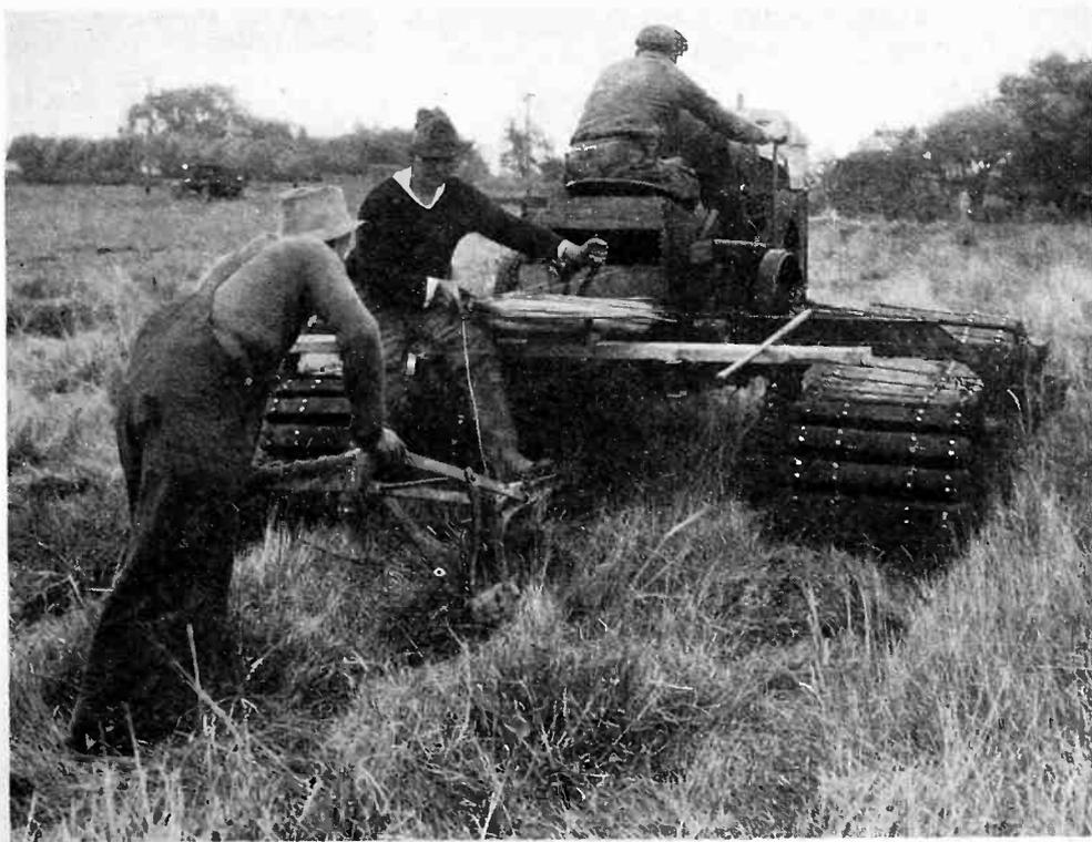
Plowing in the ground system. 35 miles of copper conductors were buried by this method, to provide the necessary ground plane
