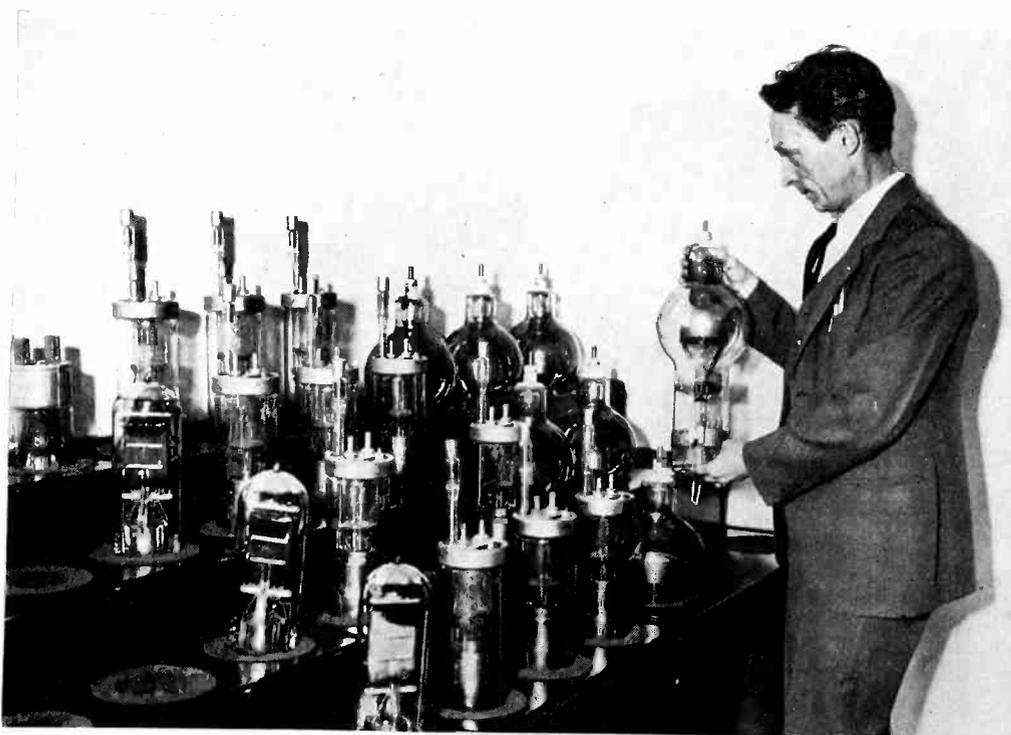
This display rack contains (left to right) 4 250-watt modulators (Western Electric type 212-E), 11 35 kw. r-f amplifiers (W. E. 232-A), and 7 10-amp. mercury rectifiers (W. E. 266-A), spares for the new 50-kw. WOR transmitter at Carteret, N. J.
