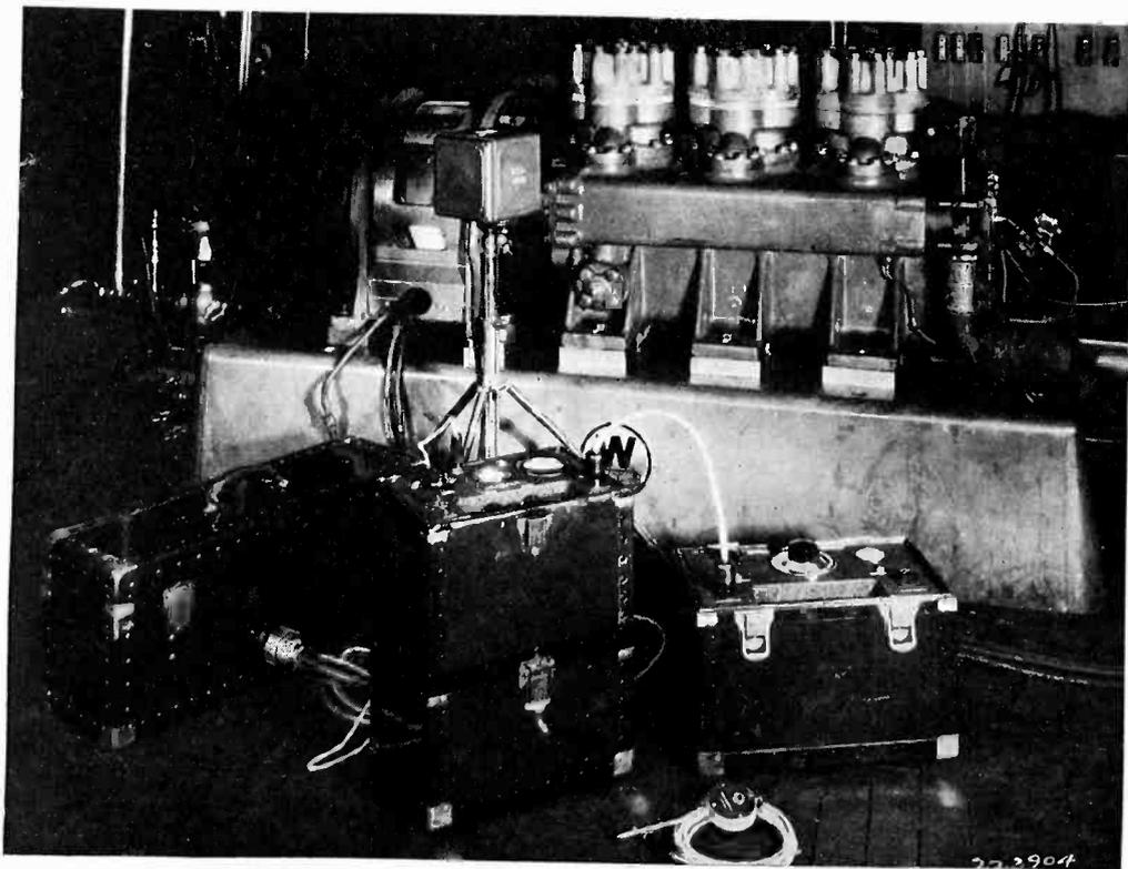
The Westinghouse noise meter and wave analyzer set up for the measurement of noise produced by a Diesel power plant. The vibration pick-up is shown in the foreground
