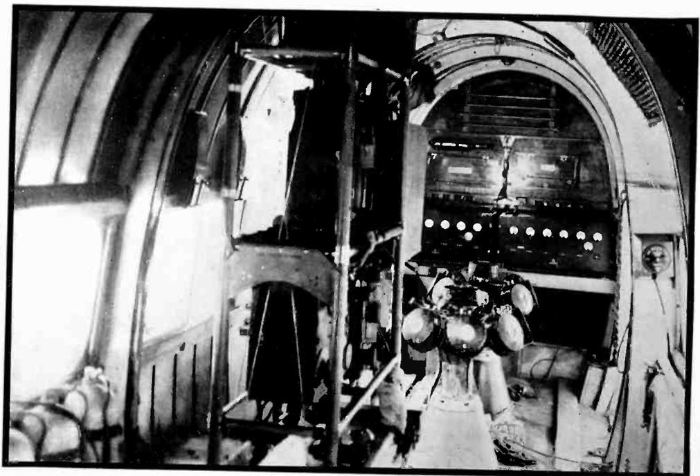
Two clusters of dynamic loudspeaker units are fitted to horns in the fuselage of this British airplane which is used in policing tribal areas in Iraq. Orders and warnings from planes seem to be much more effective than the use of force
