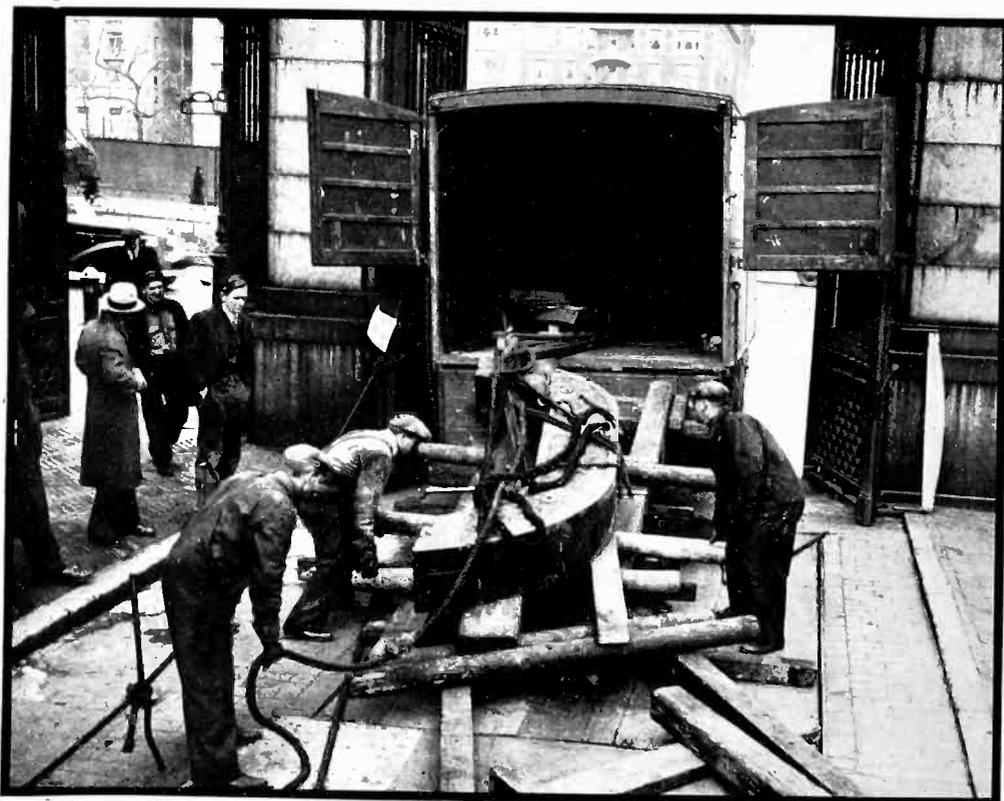
*Unloading a piece of the 130,000 pound magnet used in the arc transmitter at the Navy radio station at Annapolis until 1934, when it was replaced by vacuum tube equipment. The magnet has been given to Columbia University for use in the new 20,000,000-volt cyclotron (atomic bombardier) now under construction (see Electronics, November 1935, page 7)*
