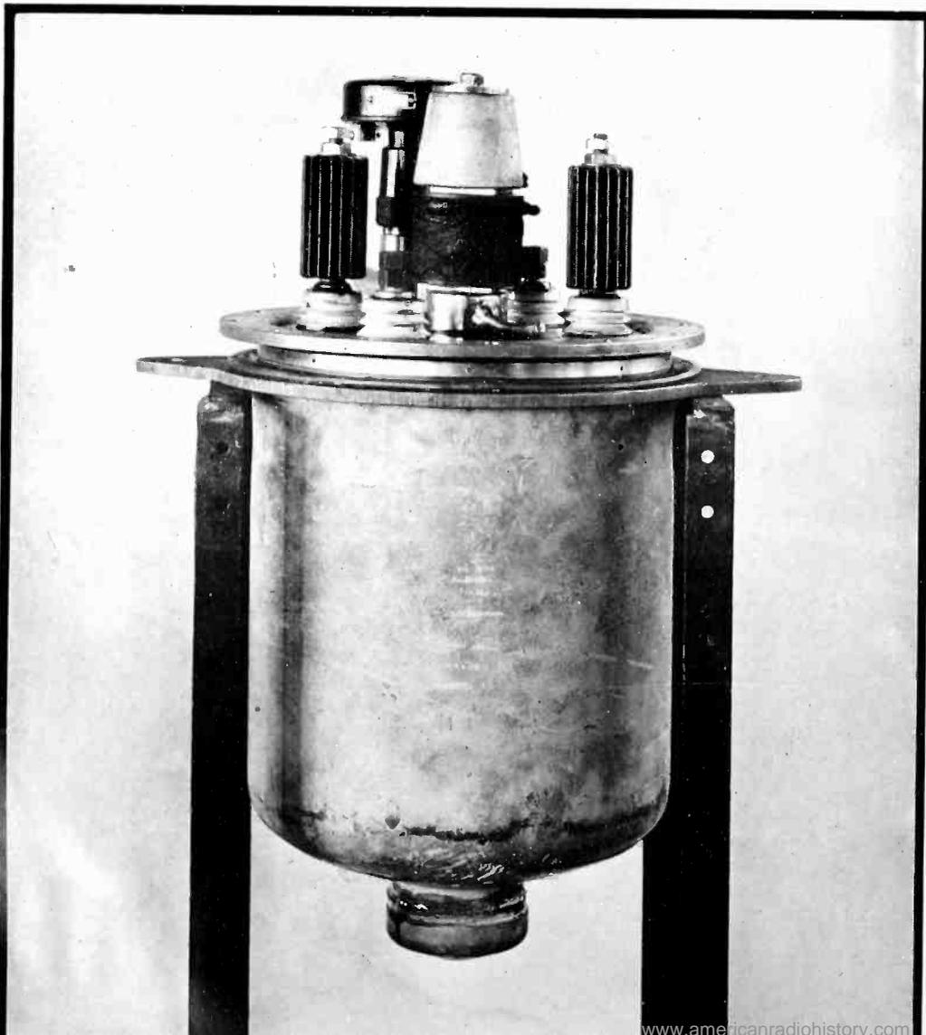
*View of the Inductotherm during the test transmission which was heard in Washington. No changes were made in the machine except to open the plate circuit for insertion of the automatic key seen on the stand at the right. The radio-frequency energy was radiated from overhead power lines after passing back through the base outlet seen just above the table leg behind the wastebasket. The call letters NDA1 were assigned to the machine for this test*
