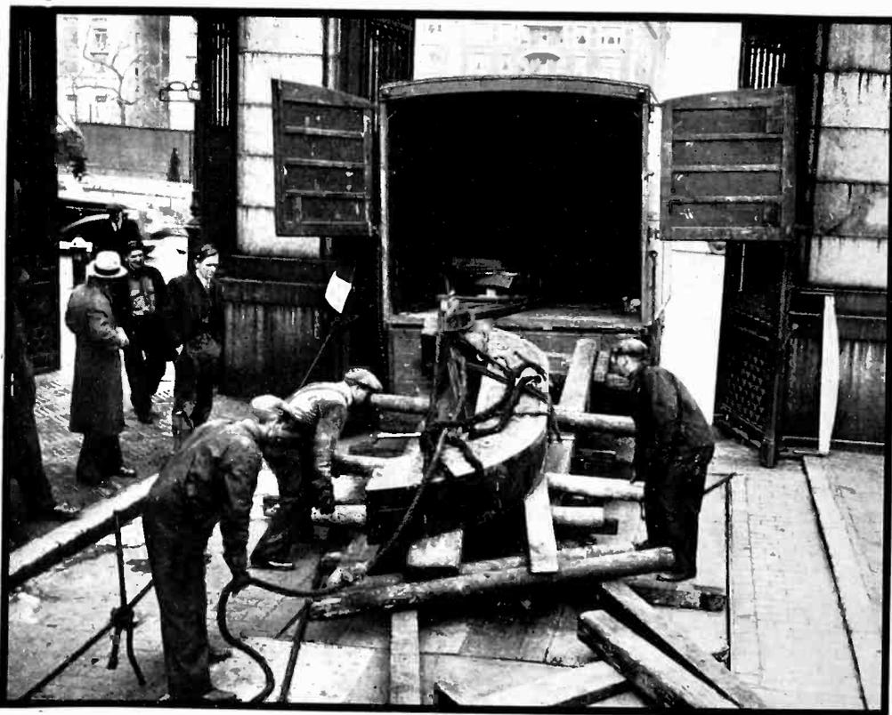
*Unloading a piece of the 130,000 pound magnet used in the arc transmitter at the Navy radio station at Annapolis until 1934, when it was replaced by vacuum tube equipment. The magnet has been given to Columbia University for use in the new 20,000,000-volt cyclotron (atomic bombardier) now under construction (see Electronics, November 1935, page 7)*
