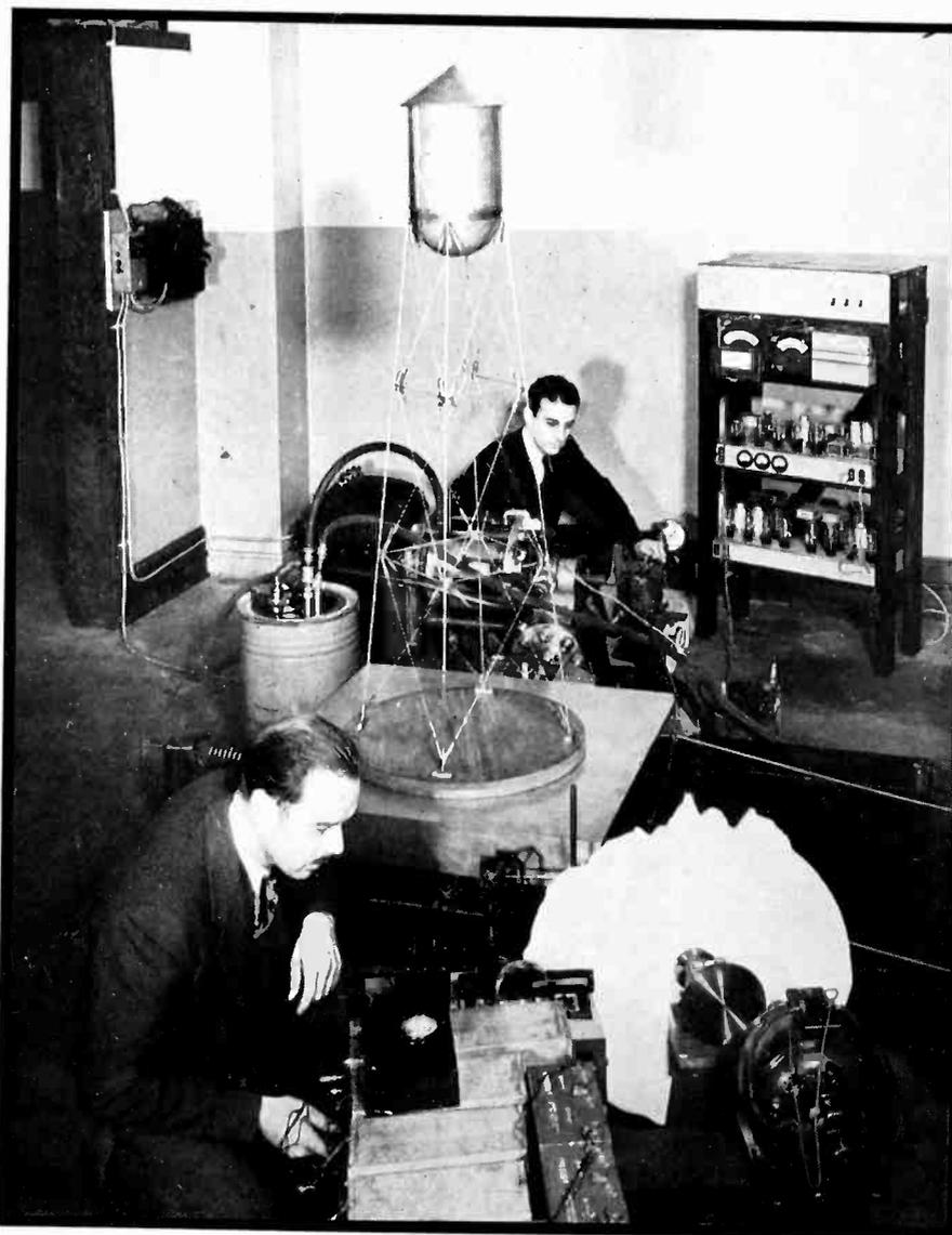
*The earthquake "shaking table." Actual earthquake records are plotted on the "optical cam" (white card, foreground) and caused to intercept light entering a photocell. The cell controls a power amplifier. This in turn controls a magnetic valve which admits oil under pressure to a piston connected to the table. The model water-tower is thus subjected to motions reproduced from actual seismic disturbances*
