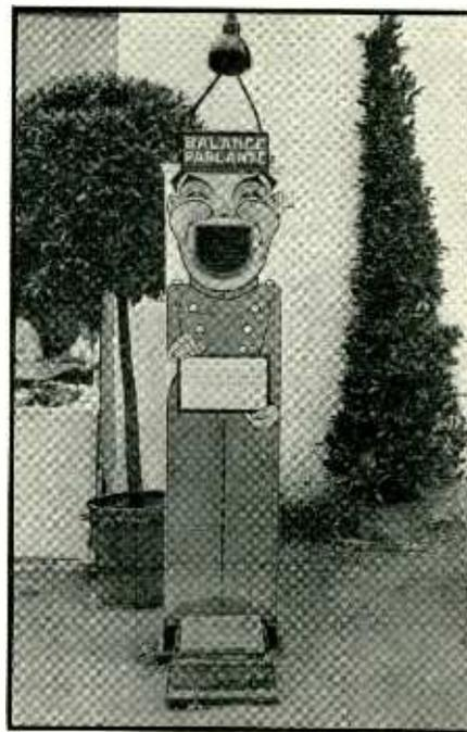
This weighing machine, recently exhibited at Brussels, announces the exact weight of the customer by means of a loudspeaker and record system
