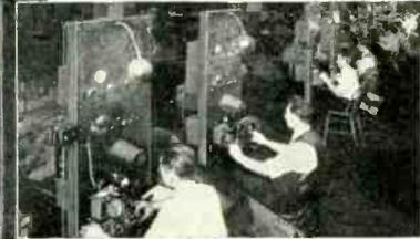
Ten Aladdin production lines using cathode-ray oscillograph testing.
